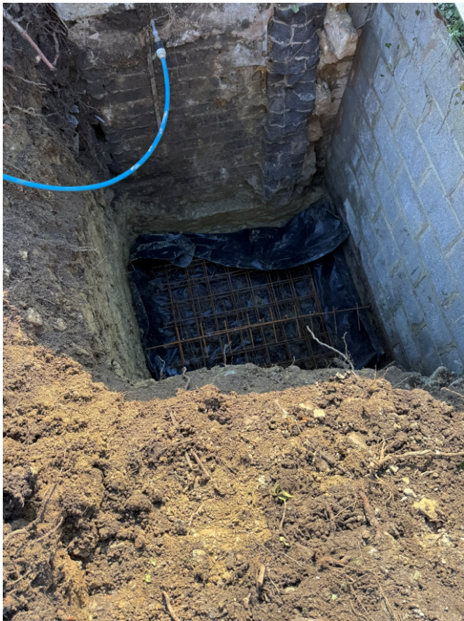
04.03.2026 Reinforcement installation
