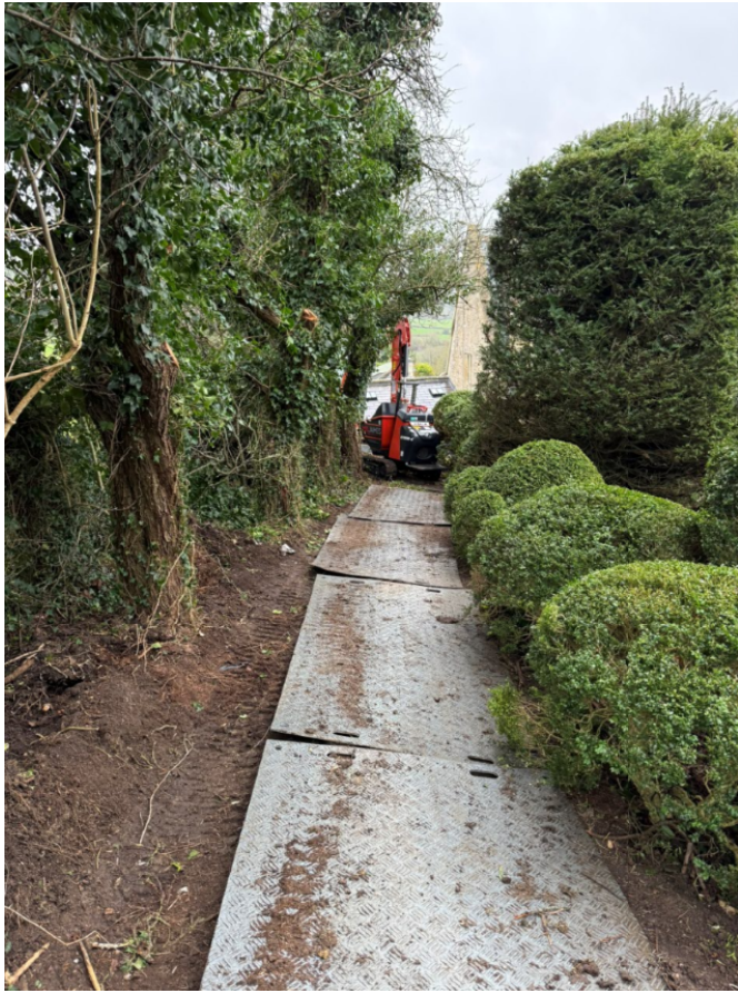
26.02.2026 Site access preparation
