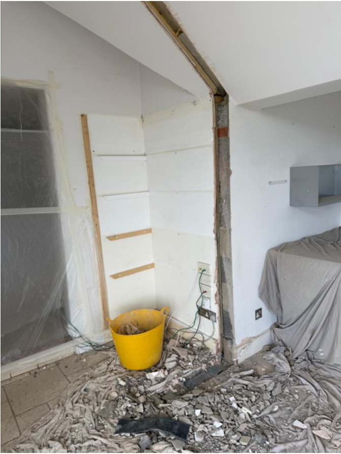
03.03.2026 Internal wall demolition
