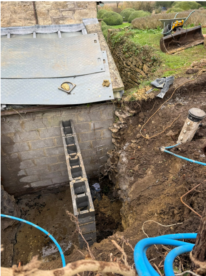
05.03.2026 Retaining wall construction
