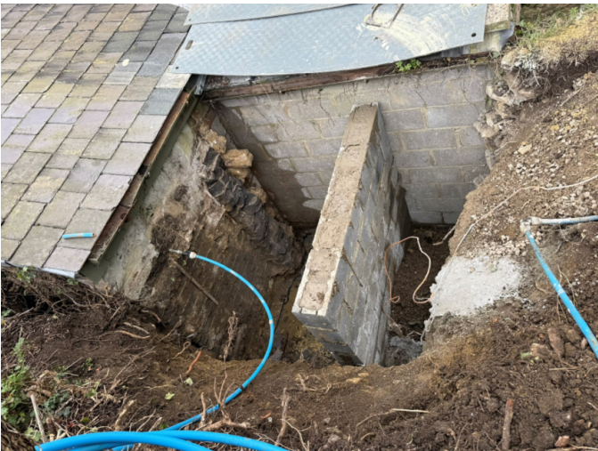
10.03.2026 Retaining wall reinforcement and concrete infill
