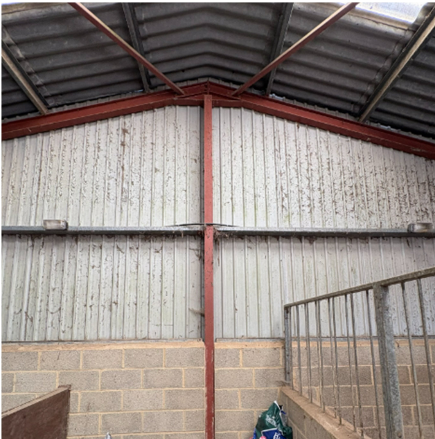
Figure 2. internal view of North gable showing central wind-post and roof bracing.
