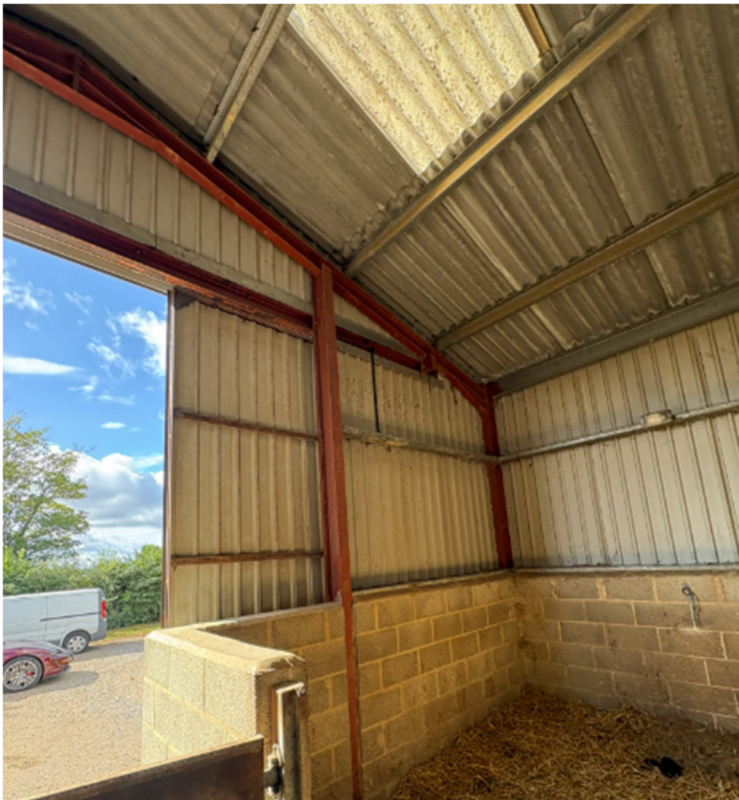
Figure 4. Front entrance on south elevation showing sliding doors and trimming steelwork around opening.
