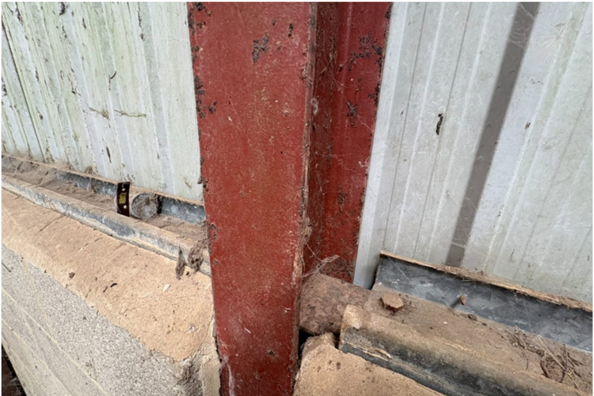
Figure 6. Typical cladding rail connection to main stanchion.
