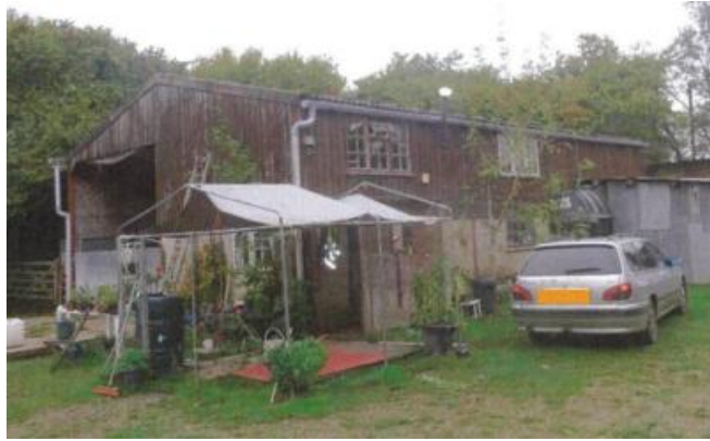
Figure 7: extract of photo from structural report
