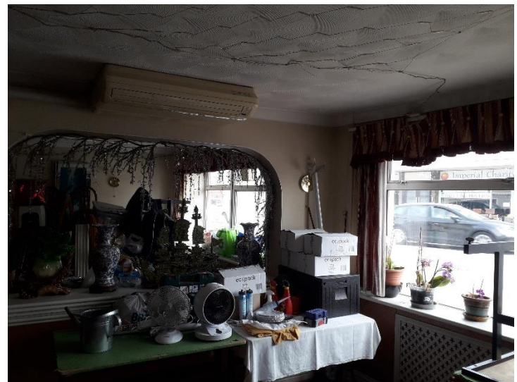
4. Application site – view to front elevation
