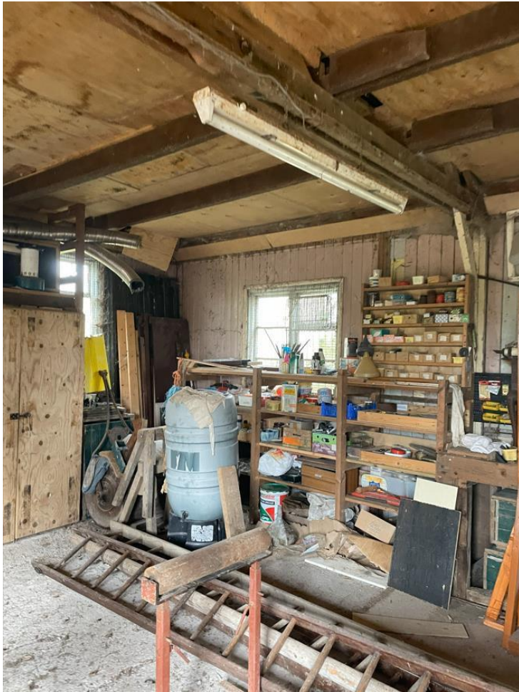
Photo showing inside of builders workshop (Acorus Rural Property Services Ltd)
