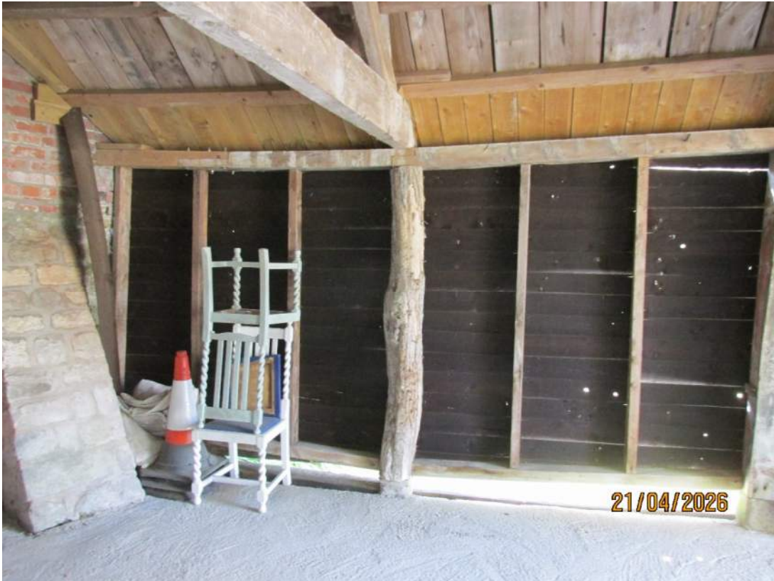
Building 2 – Internal view of posts supporting timber A Frame roof trusses
