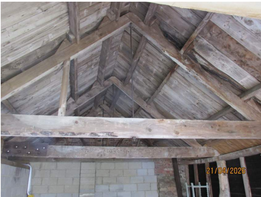
Building 2 – Internal view of roof, end gable (party) wall and timber framed wall to south
