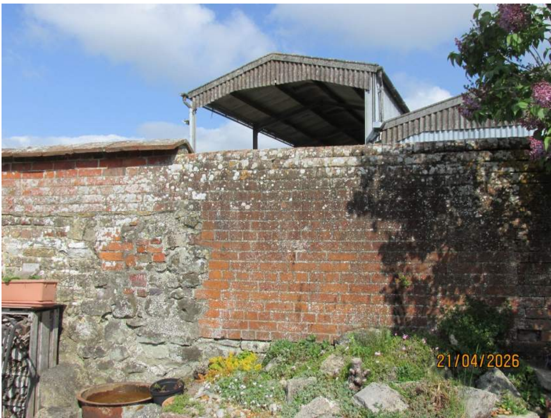
Building 2 – View of boundary party wall along which extension is proposed
