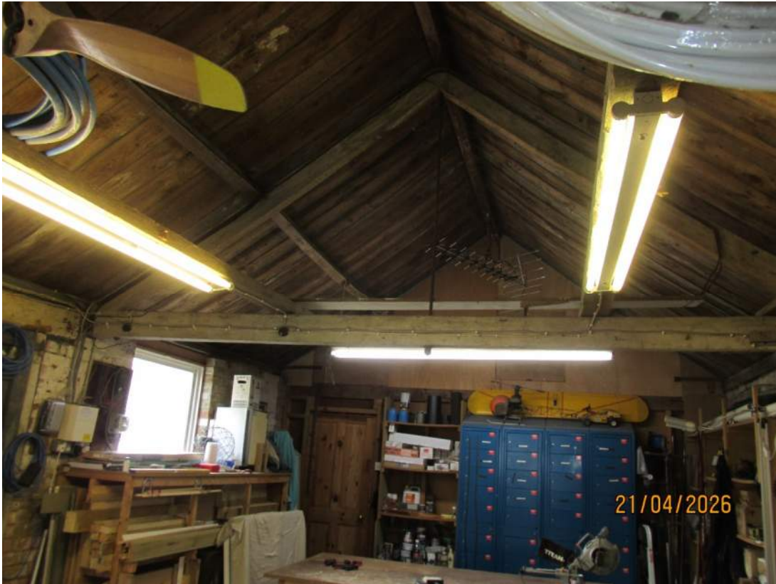
Building 1 - Internal view of Workshop showing roof construction
