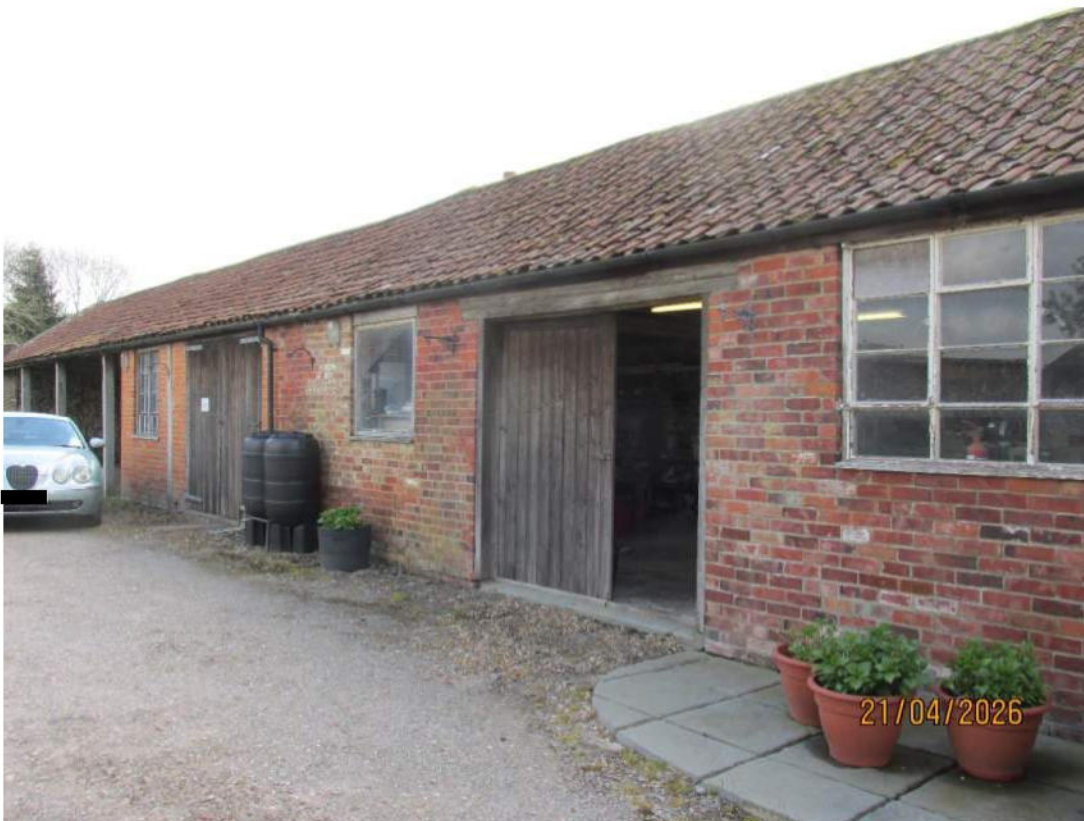
Building 1 - External 'front' elevation
