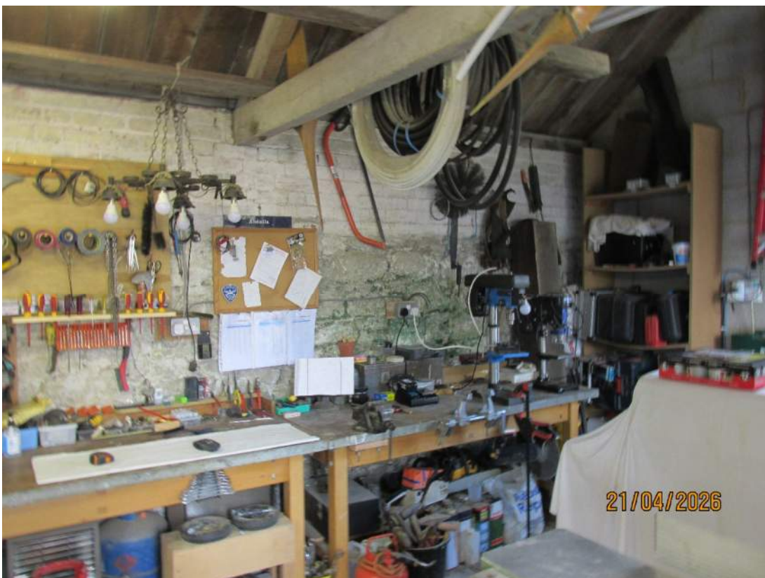
Building 1 – Internal view of rear party wall supporting roof
