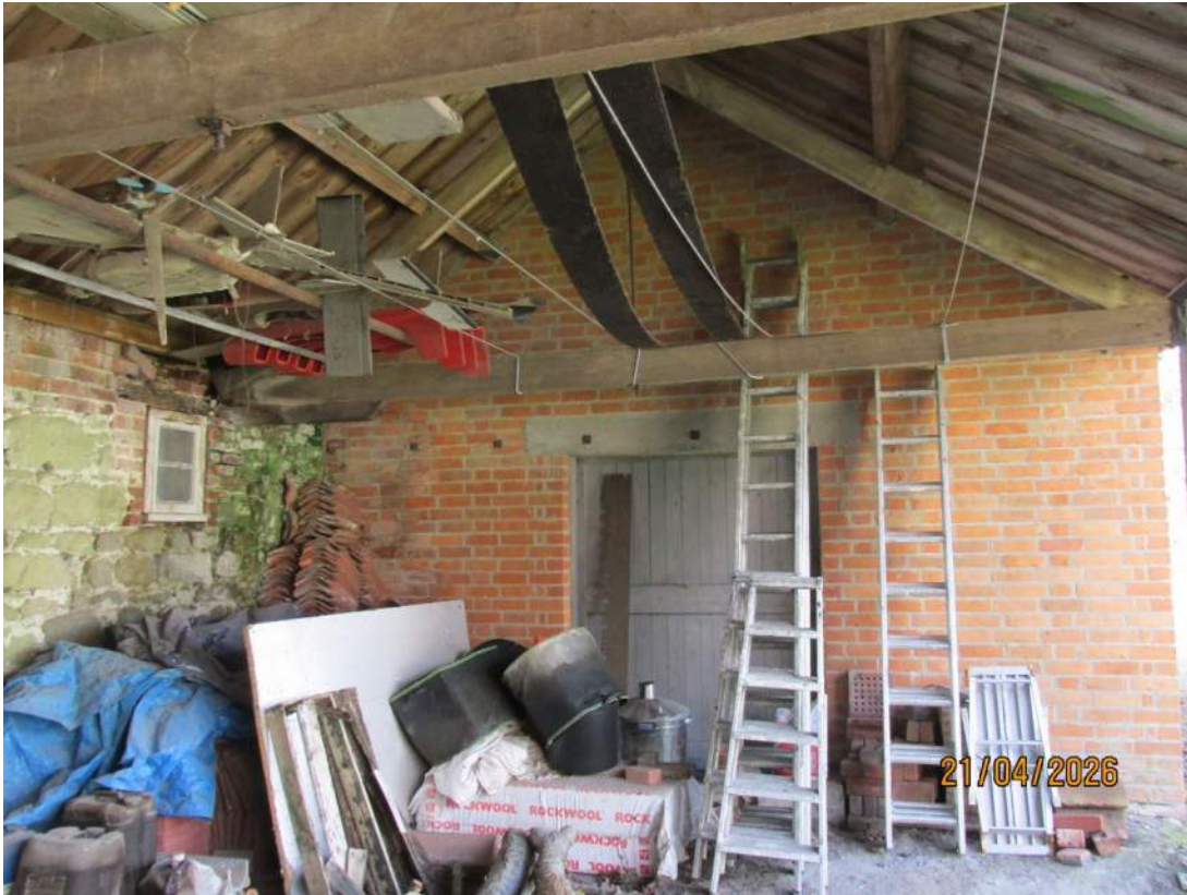
Building 1 – Masonry gable wall between Sewing Room and open fronted Store
