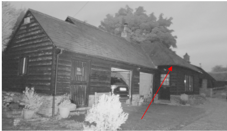
Photograph 2: Roost 1 exit location.
