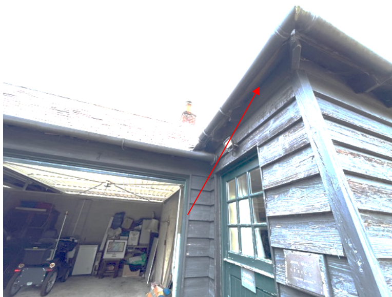
Photograph 1: Roost 1 exit location.
