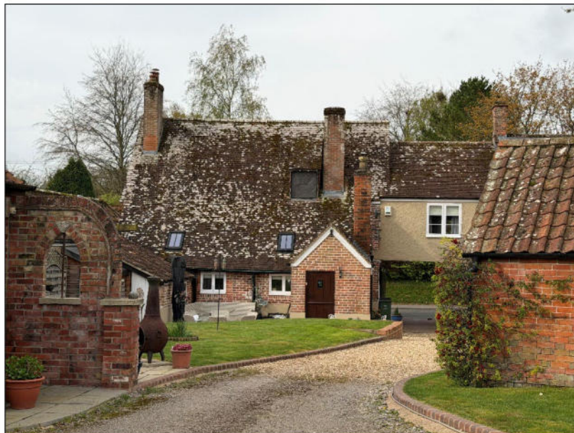
Image 17: No. 69 High Street, rear elevation
