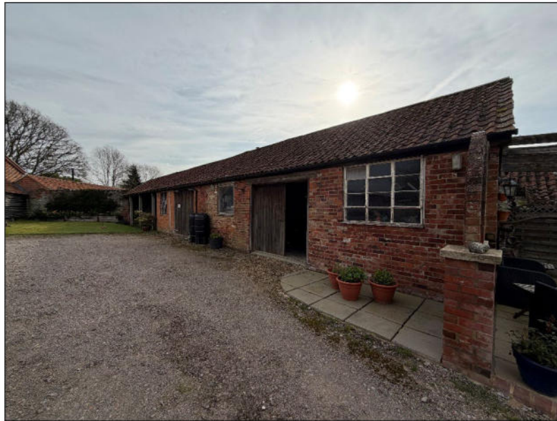
Image 13: Outbuilding viewed from southwest
