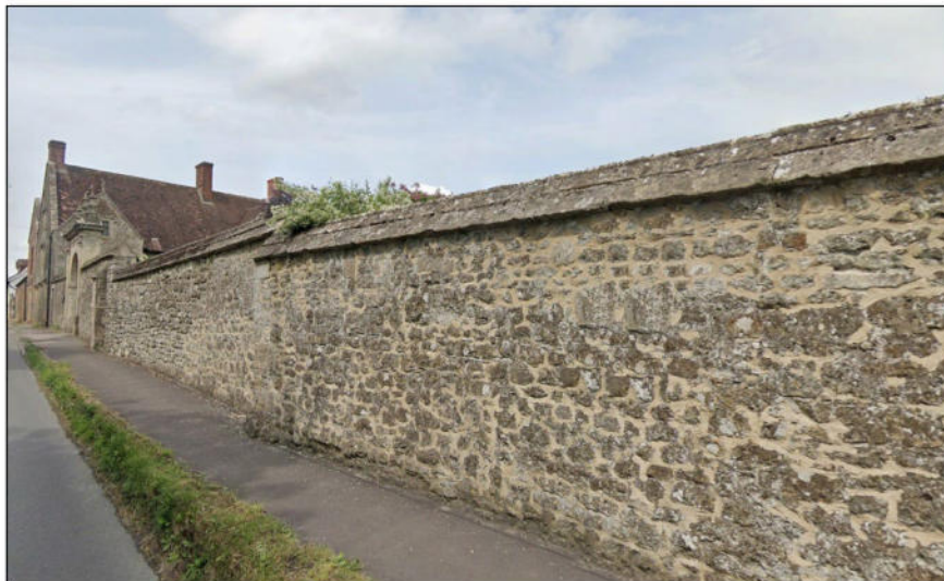
Image 19: Boundary wall to West Lavington Manor
