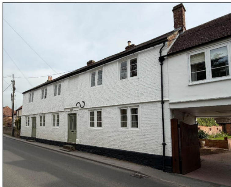
Image 20: Nos. 63 and 65 High Street, front elevation
