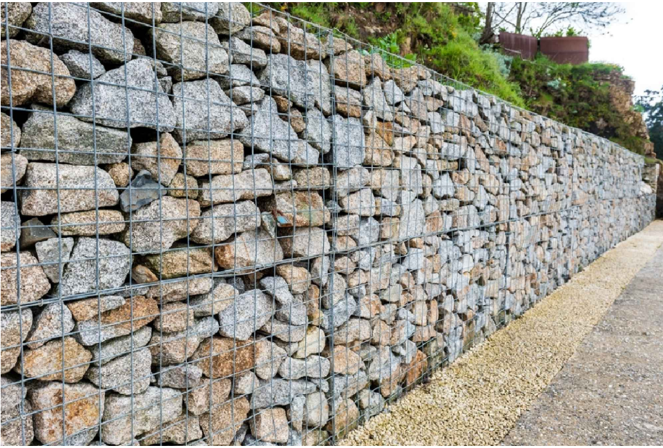
Example of Gabion Retaining Structure
