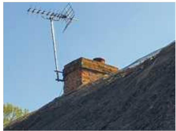
Figure 4: The west and south elevations of the chimney stack
