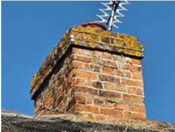
Figure 5: The south and east elevations of the chimney. The mortar cavities could be fully inspected from the ground using binoculars which confirmed shallow cavity spaces
