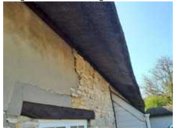
Figure 2: The eave of the west elevation showing an example of the wire mesh which is in good condition throughout the roof
