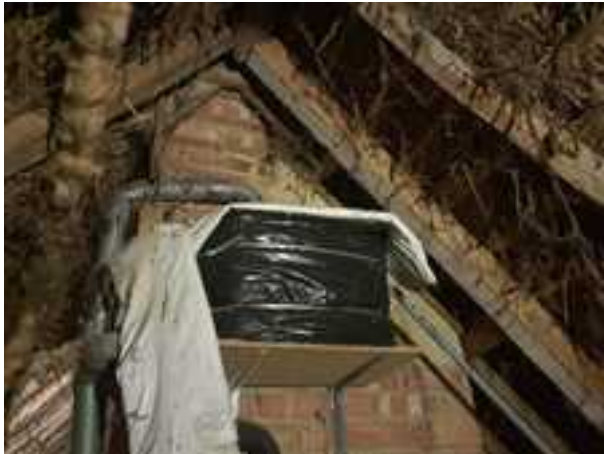
Figure 7: The south elevation of the chimney breast within the loft void
