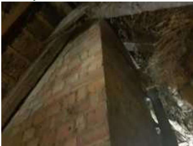
Figure 9: The north and west elevations of the chimney breast
