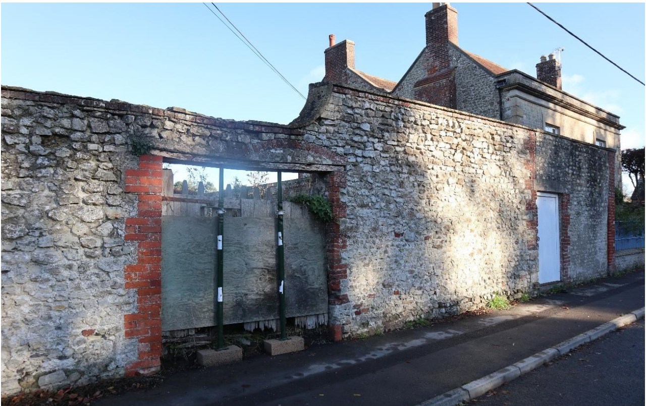
Figure 1 The LBC application site comprising the Boreham Road Boundary wall to the west of The Cotes (Grade II).
