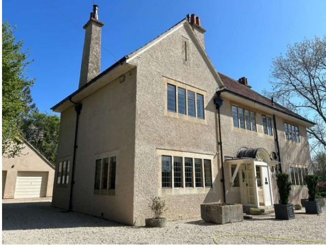
Photo 1: Southern and western elevations of B1.
