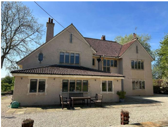
Photo 3: Northern elevation of B1.
