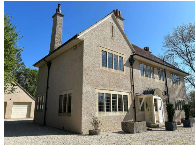
Southern and western elevations of B1.
