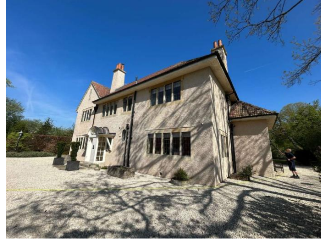
Photo 2: Southern and eastern elevations of B1.
