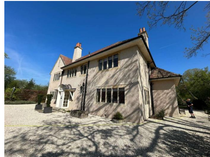
Southern and eastern elevations of B1.
