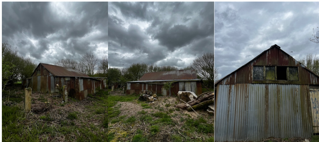
Figure 8. Visual overview of the structure (left – north, centre – west, right – south)
