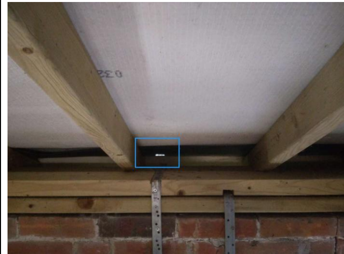
B2 - Gaps along the verge in the loft
