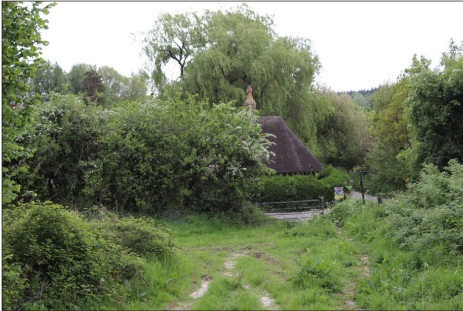
Plate 7: The roof of Turnpike Cottage looking south from the footpath north of Smallbrook Road
