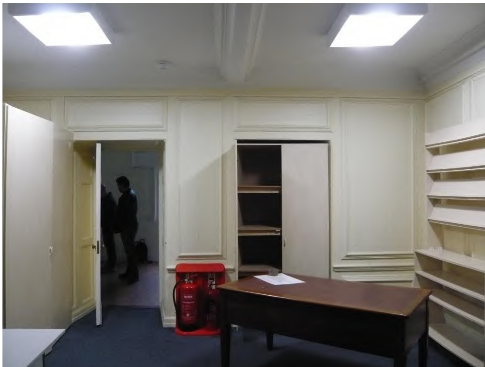
Fig.11 Ground floor front room with full-height C18 panelling
