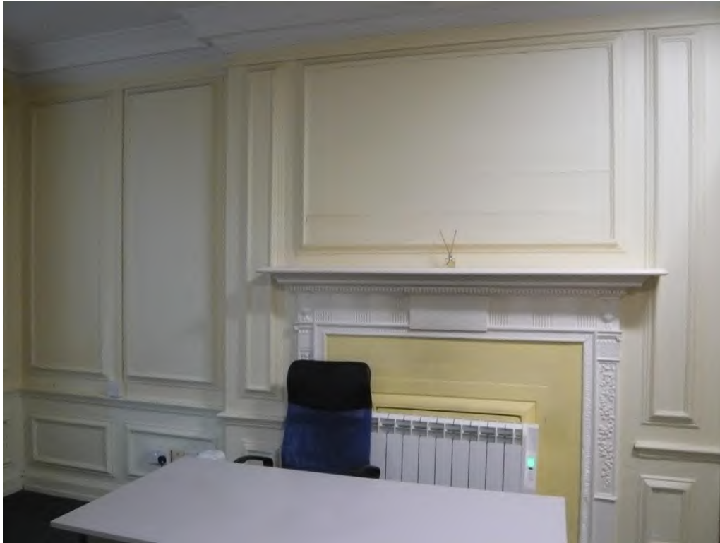
Fig.12 Fireplace on east wall of ground floor front room
