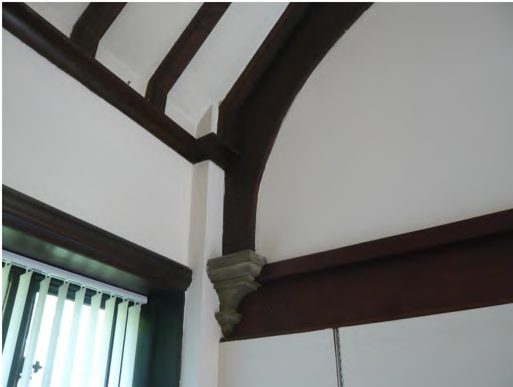
Fig.27 Exposed collar beam truss on stone wall posts within W Range
