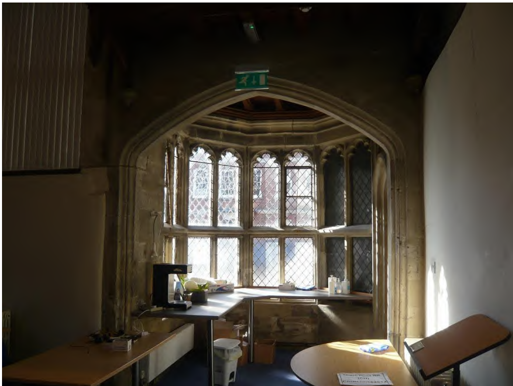
Fig.7 Bay window at S side of hall
