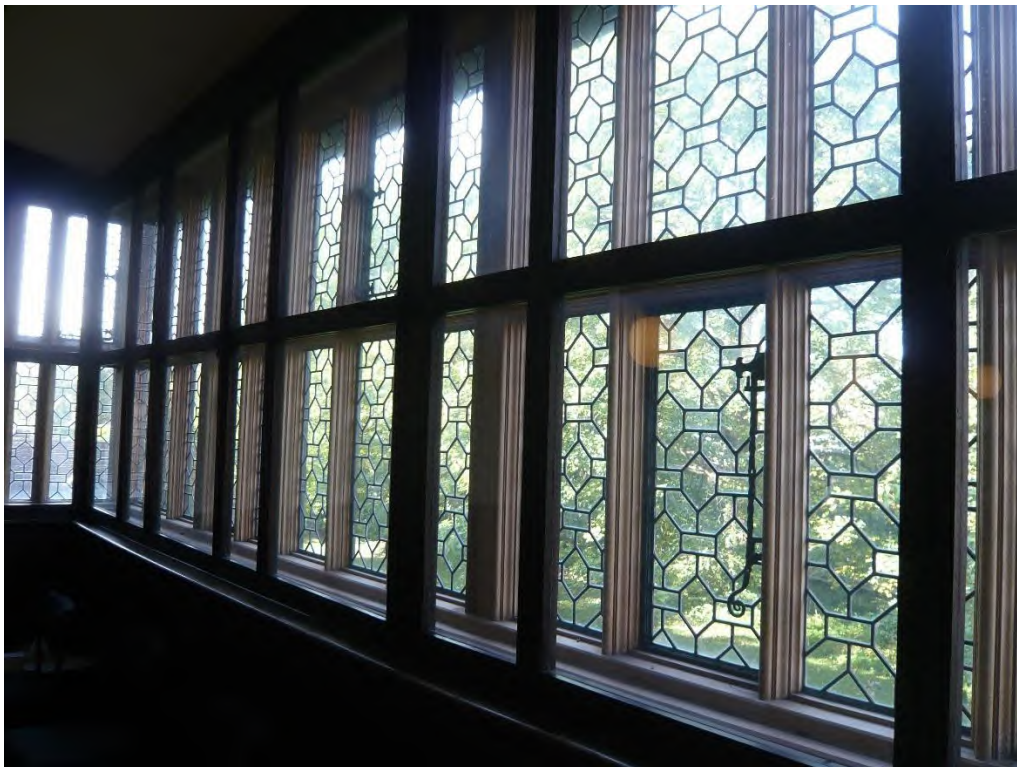
Fig.11 C16 transomed and mullioned window in board room
