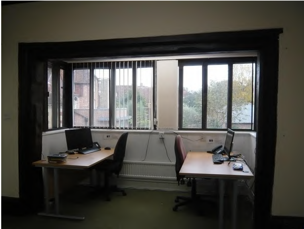
Fig.28 C16 architrave and linings to bay projection in centre of W Range
