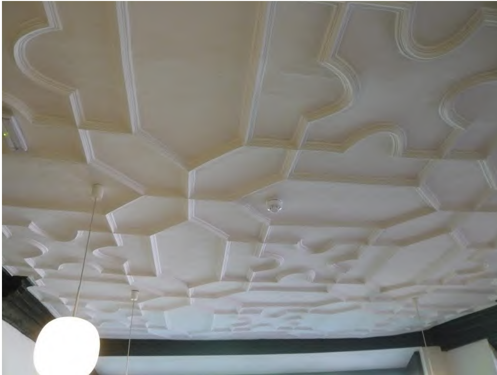
Fig.10 C16 ribbed plaster ceiling in board room
