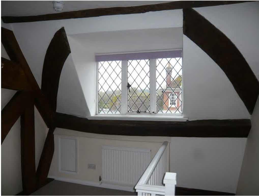
Fig.20 Dormer cut through C15 arched braces at western end
