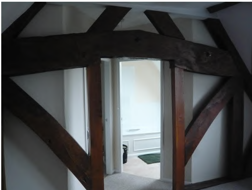
Fig.19 Doorway formed through western C15 truss, modern bathroom partitions beyond
