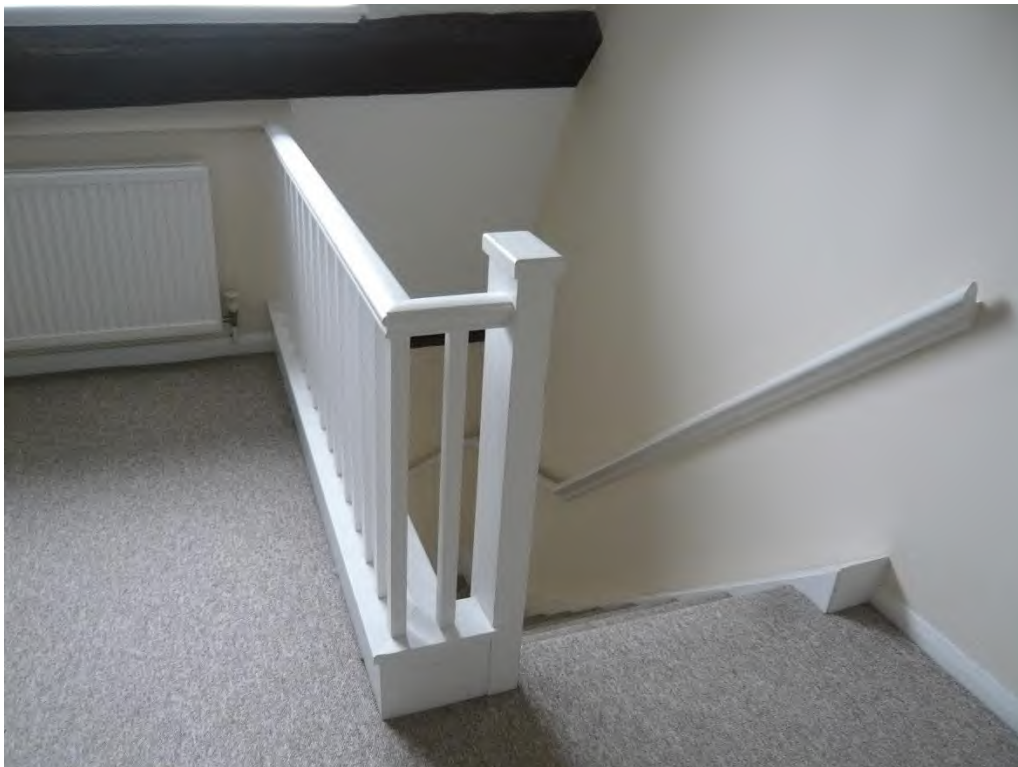
Fig.21 Modern staircase serving the second floor
