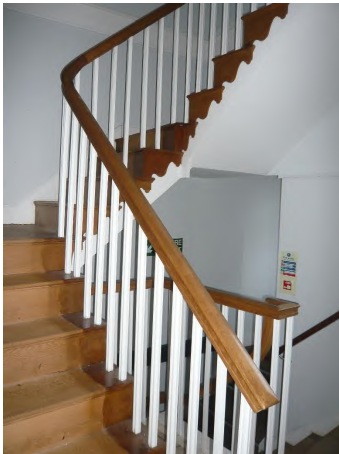
Fig.39 1969 staircase to second floor flat
