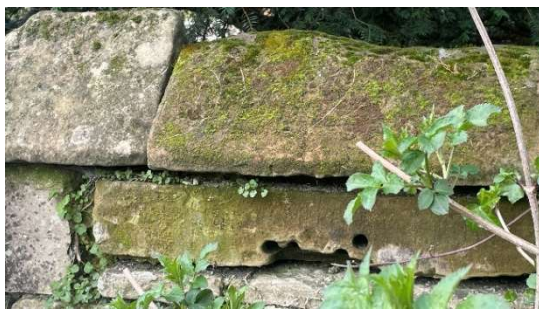
Figure 3.16c: Missing pointing
