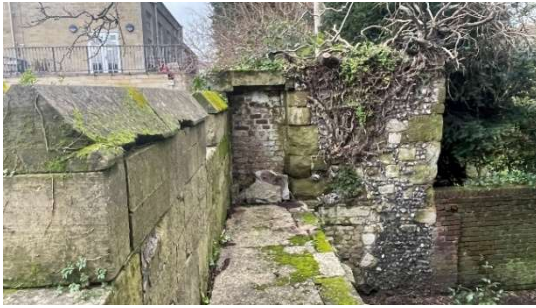
Figure 3.9e: The wall walk looking east
