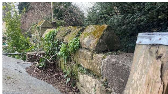
Figure 3.16b: The lower parapet facing no. 3/5
