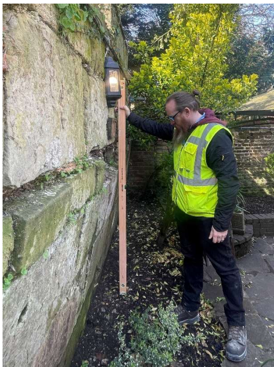
Figure 3.13b: The extent of lean to the north is alarming
