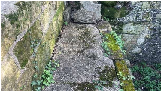
Figure 3.9g: Wall walk concrete capping
