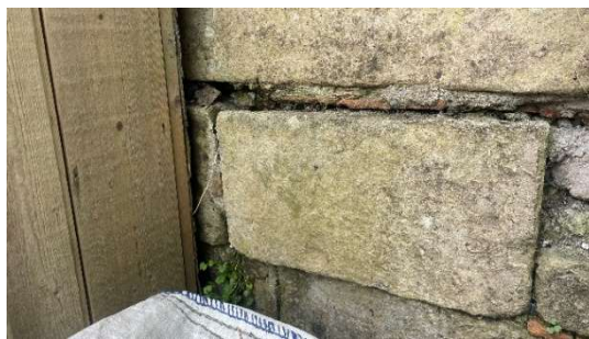
Figure 3.16d: Stone to be re-set
