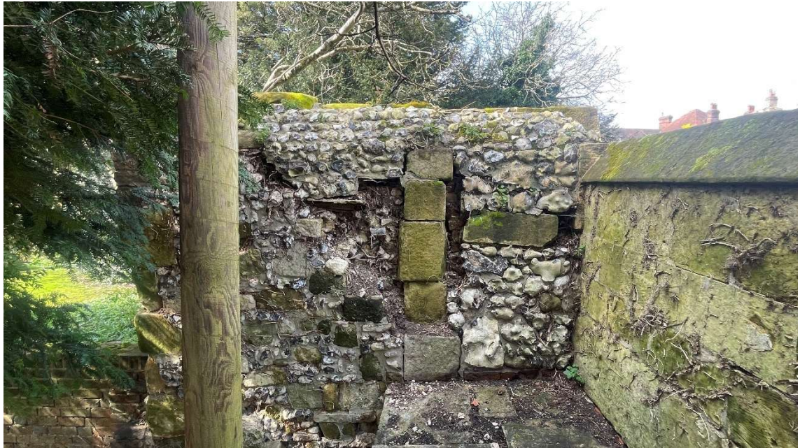
Figure 3.6a: The south return wall between nos 18 and 17 from the east
