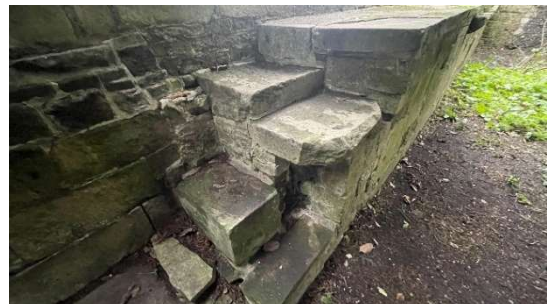
Figure 3.9d: Ad-hoc steps (non-original)
