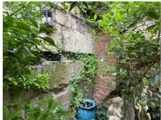
Figure 3.14b: Junction with Party wall to west of No. 1
