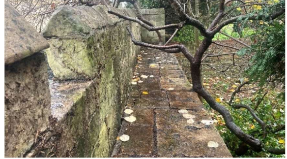
Figure 3.2d: Wall walk looking east
