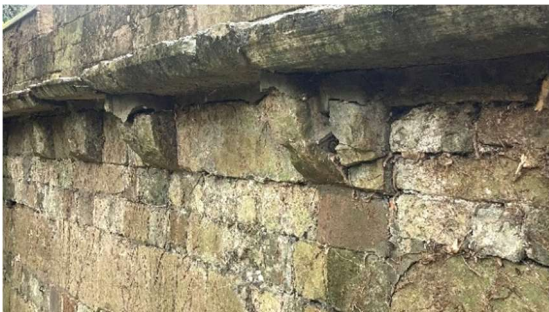
Figure 3.2a: Stone corbels supporting the wall walk
