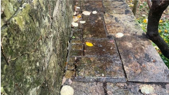
Figure 3.2e: Wall walk paving
