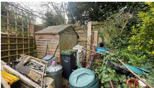
Figure 3.16a: The wall to no. 3/5 is difficult to access
