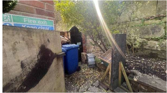
Figure 3.15b: The area to be lowered (under the crate)
