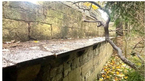
Figure 3.2b: The wall walk
