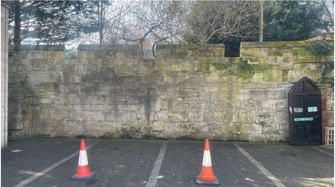
Figure 3.7a: The north face of the wall from the car park of Alexandra House
