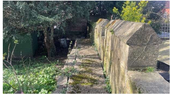
Figure 3.9h: The crenellated parapet
