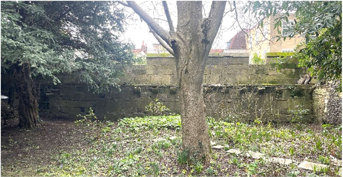
Figure 3.9: The south face of wall in the garden of no. 18 The Close
