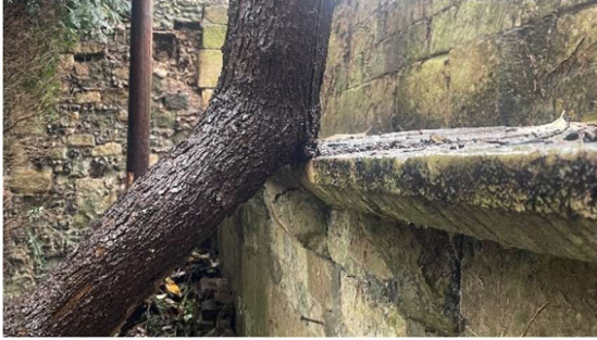
Figure 3.2c: Branch growing into the wall walk
