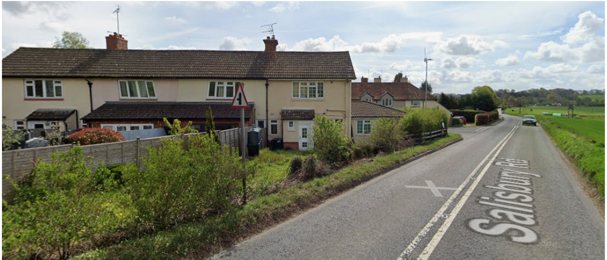
Existing residential housing (north) – Salisbury Road, leading to Thorne Road
