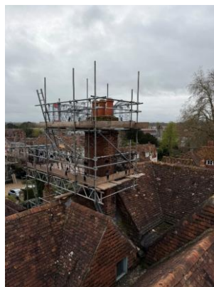
Figure 33 – View from Chimney A
