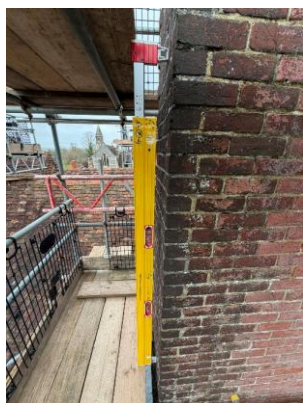
Figure 24 – South verticality check
