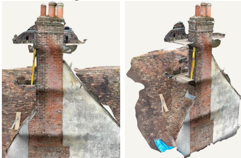
Figure 15 – Chimney B LiDAR scan images [L-R = east, SE]
