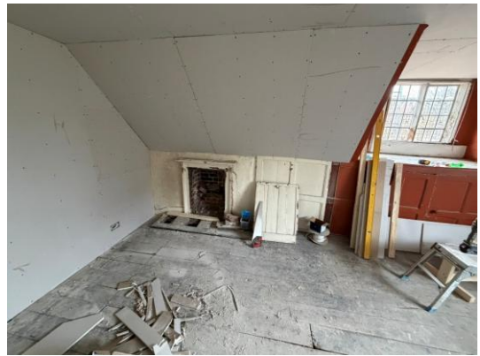
Figure 50 – Internal, top floor
