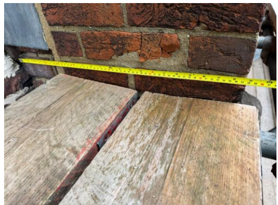
Figure 52 – South elevation measurement
