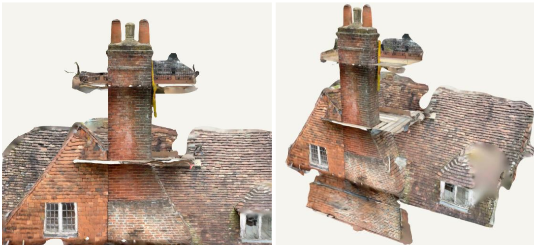
Figure 6 – Chimney A LiDAR scan images [L-R = west, SW]
