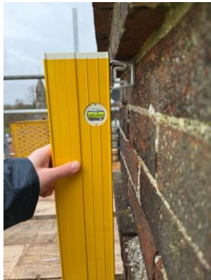
Figure 11 – South verticality check
