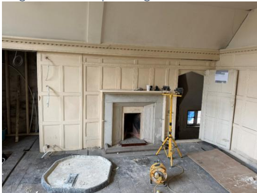
Figure 30 – Internal, top floor
