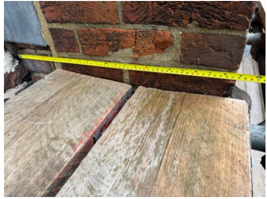
Figure 48 – South elevation measurement
