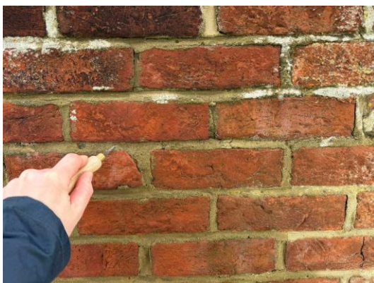
Figure 41 – Cement pointing at north
