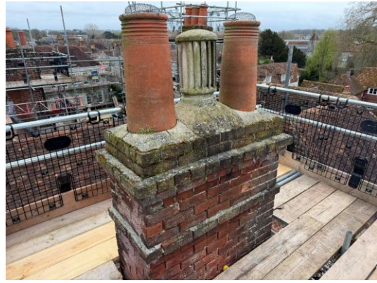
Figure 10 – Looking south east across roof
