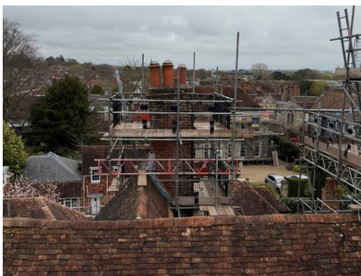
Figure 16 – View from Chimney A
