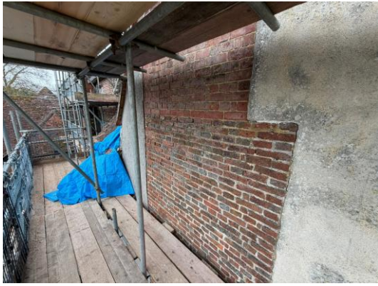
Figure 18 – East elevation within gable
