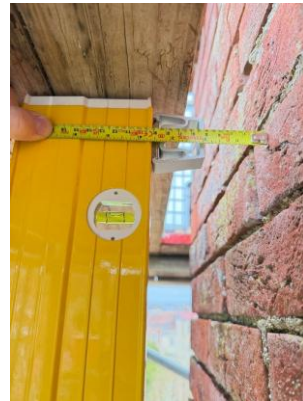
Figure 12 – West verticality check
