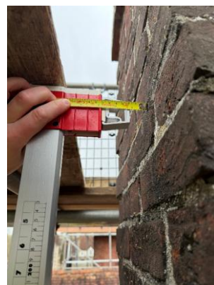
Figure 25 – East verticality check
