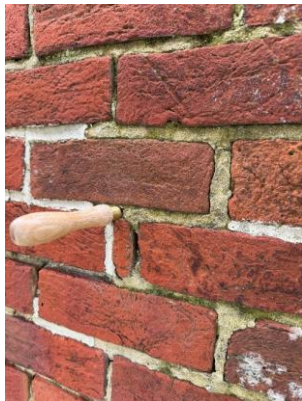
Figure 28 – Soft pointing on east elevation
