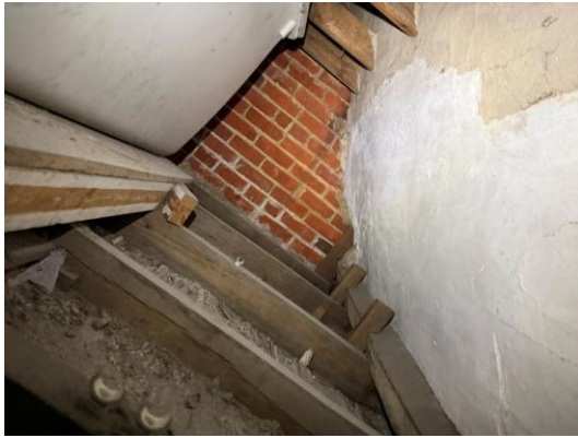
Figure 43 – Base of stack within roof
