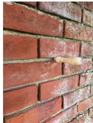
Figure 14 – Penetration with bradawl
