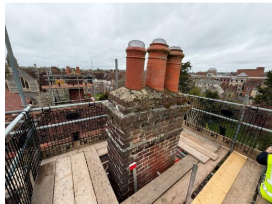
Figure 21 – Top of stack looking north west
