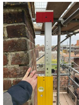
Figure 40 – North verticality check
