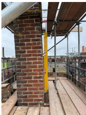
Figure 39 – North verticality check
