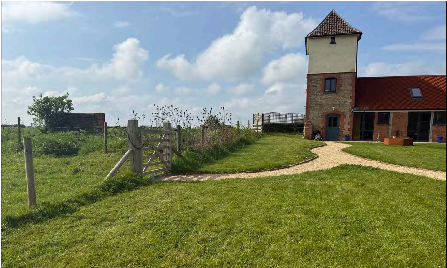
PHOTO 6 - VIEW TO WATER TOWER FROM THE SOUTH
