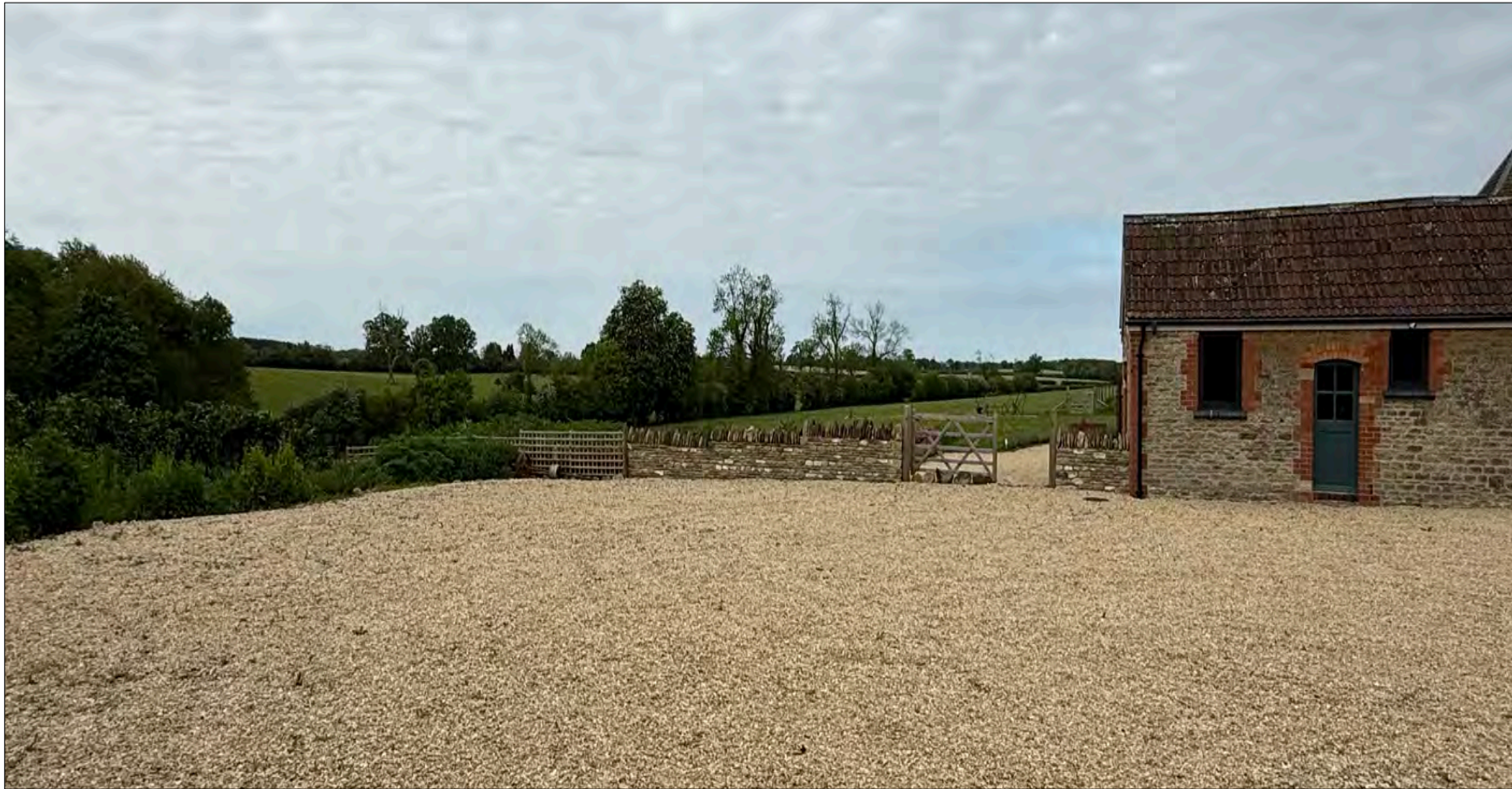
PHOTO 5 - VIEW OF COTSWOLD STONE WALL FROM PARKING AREA
