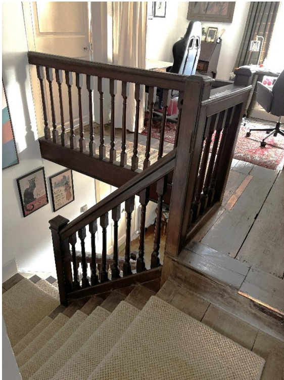
Fig. 16 Open-well stair at first floor
