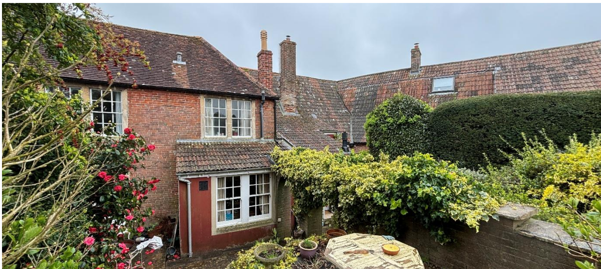
Fig. 15 Rear elevations showing tall kitchen chimney and
