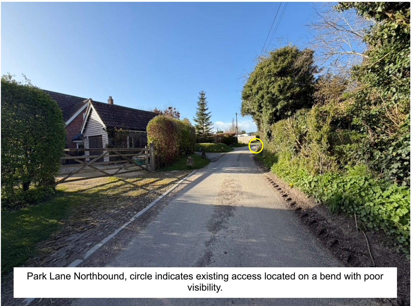
Park Lane, existing 'Right of Way' access, narrow 3.5m width, located on a bend with poor visibility.
