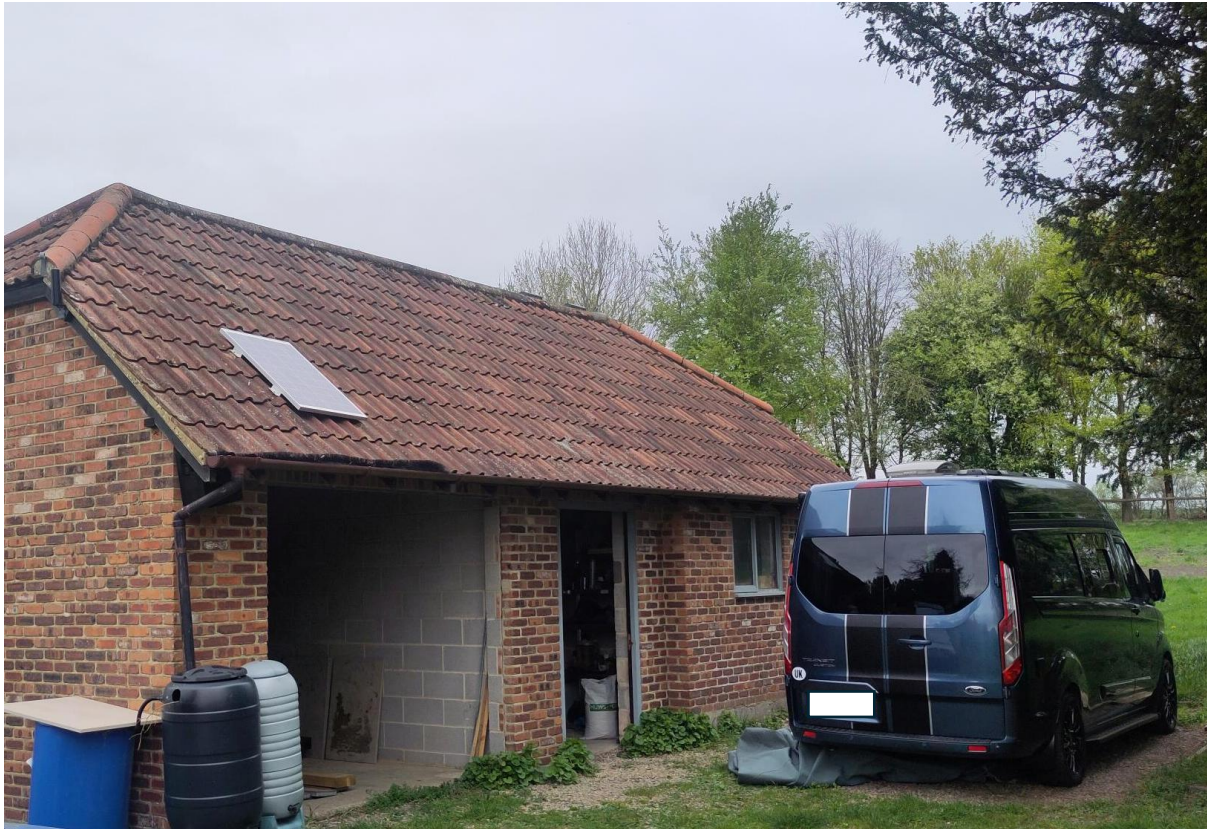
Photograph 3: showing a view of the building (facing north-east)
