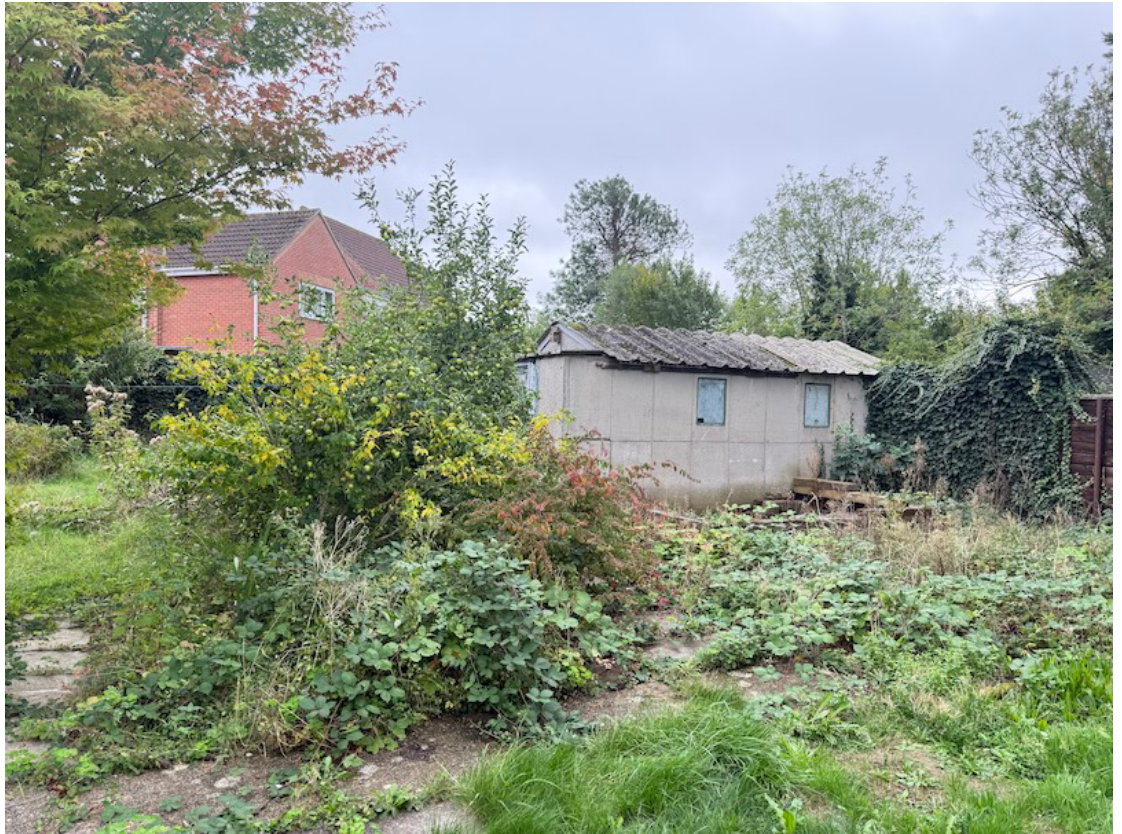
Figure 5 – View Towards Garages
