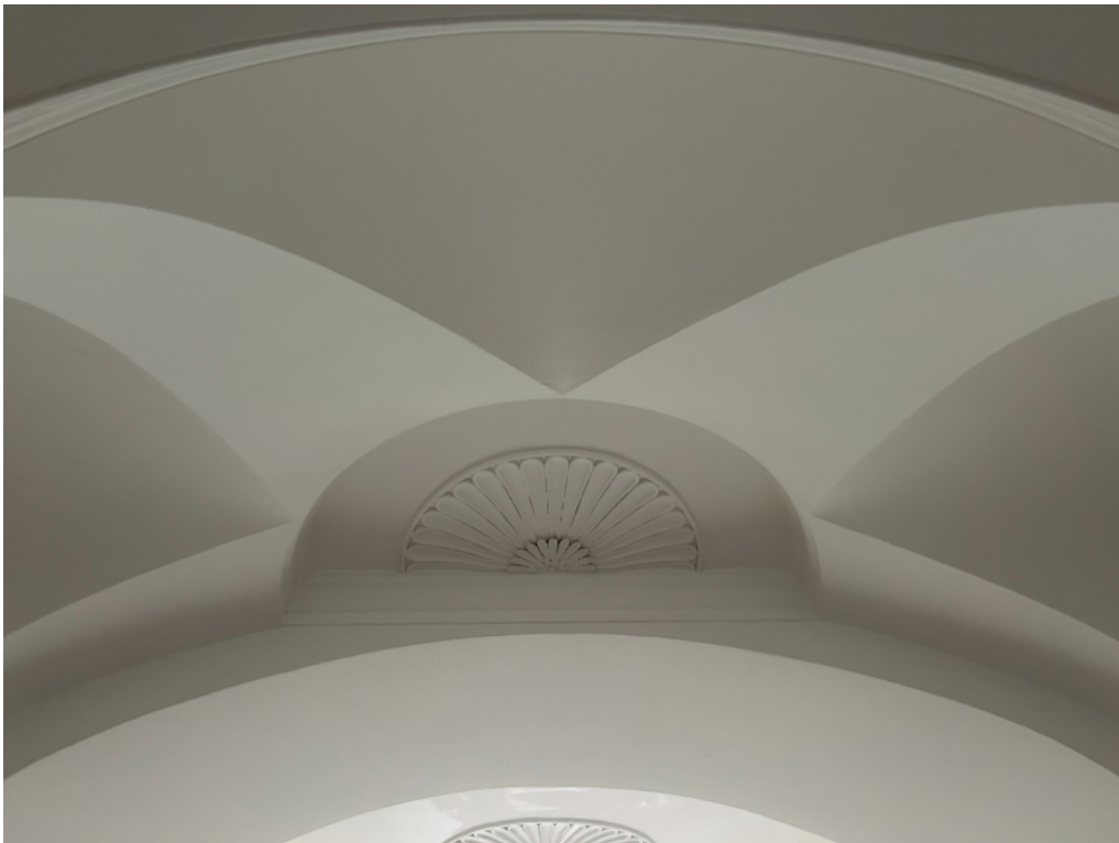
Figure 59: R.G.18, North Lobby (proposed R.G.19, North Lobby)
