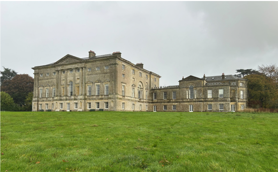
Figures 134 & 135: External, South façade
