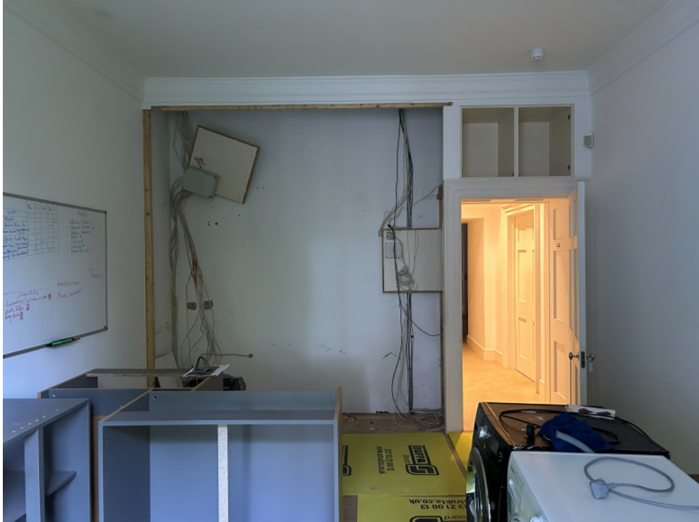
Figure 50: R.G.13, Bed 4 (proposed Laundry), door to Corridor
