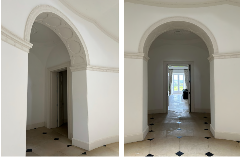
Figures 67 & 68: R.G.20, South Lobby, doorways to West Ambulatory & Garden Room
