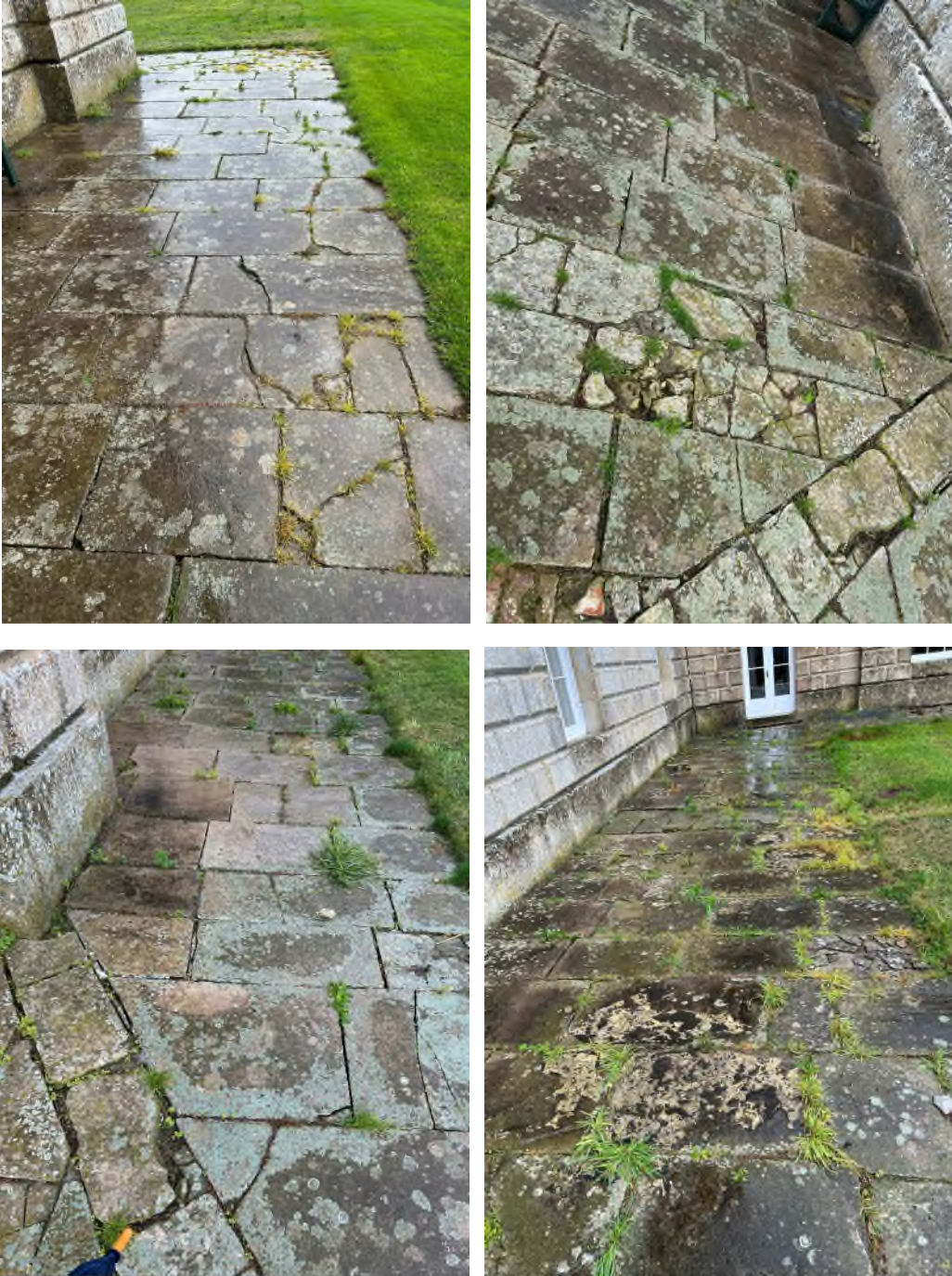
Figures 149 – 152: External, paving
