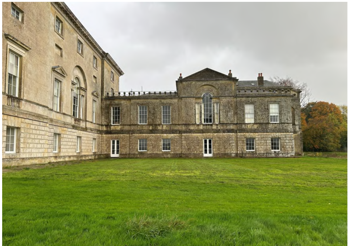
Figures 136 & 137: External, South façade, East and West wings
