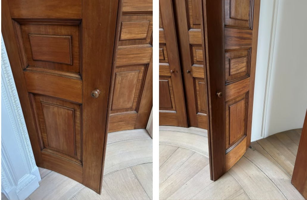
Figures 128 & 129: R.1.12, Gallery, curved double doors onto lobby
