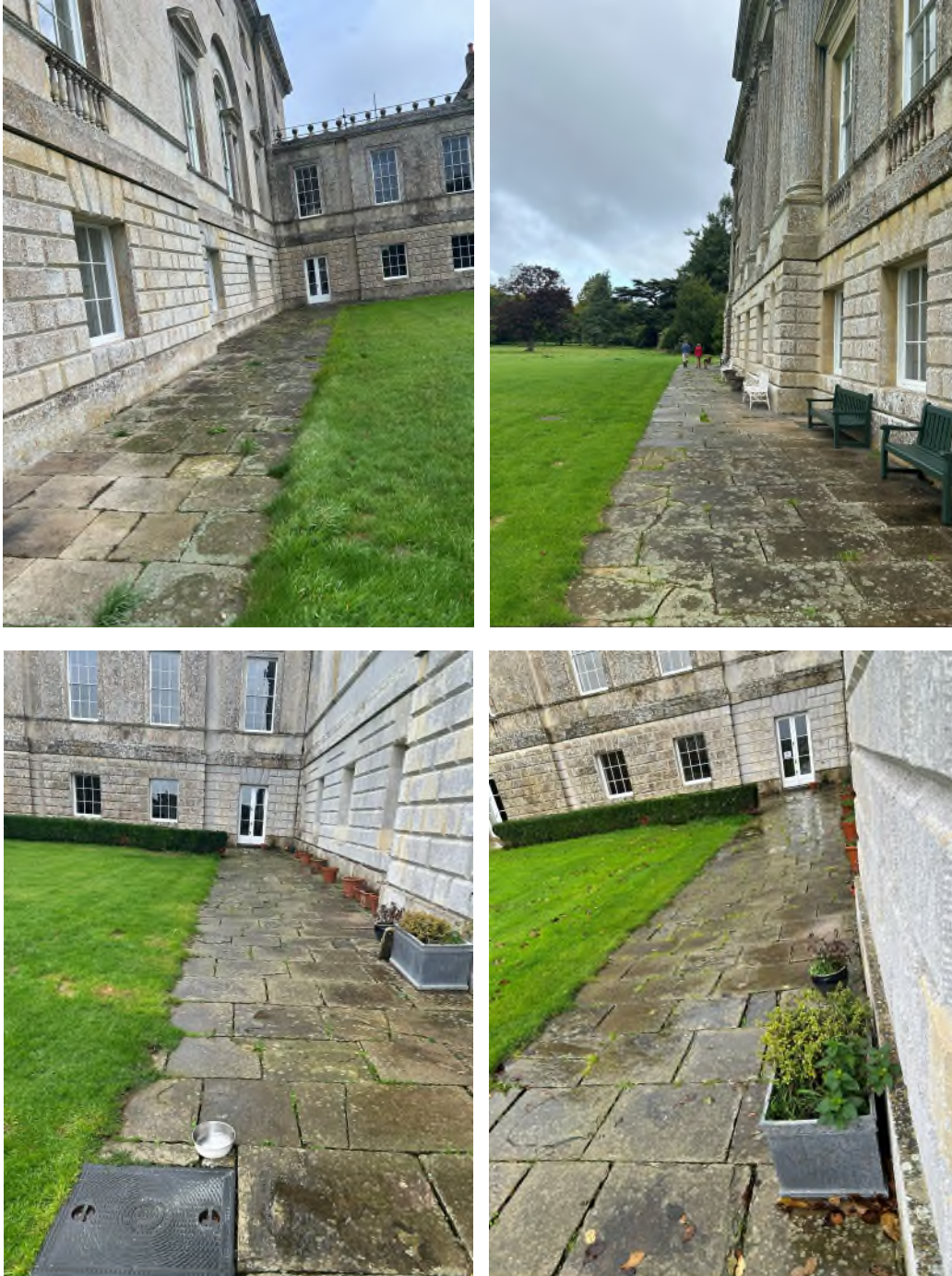
Figures 141 – 144: External, paving
