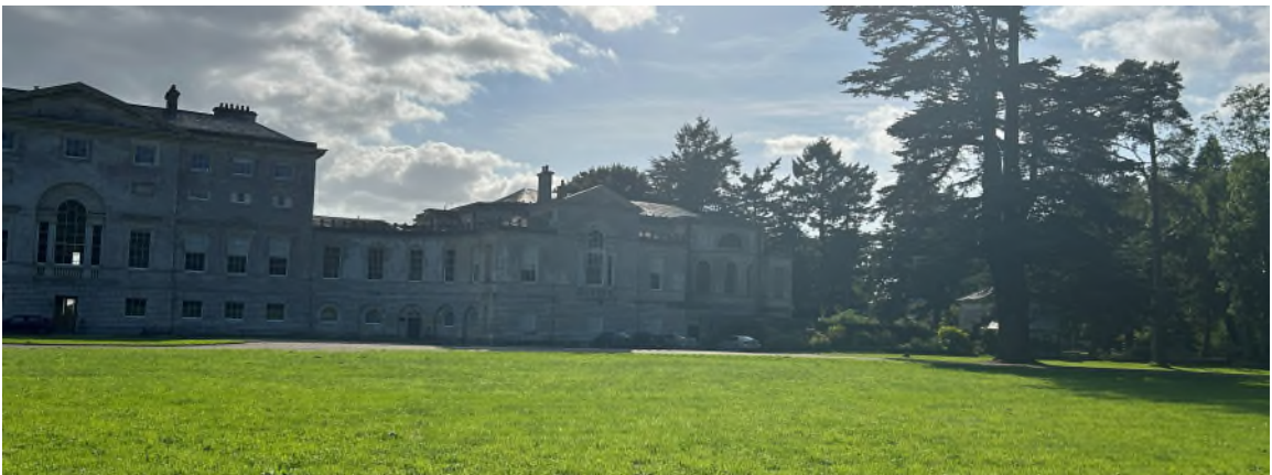
Figures 131 – 133: External, North façade
