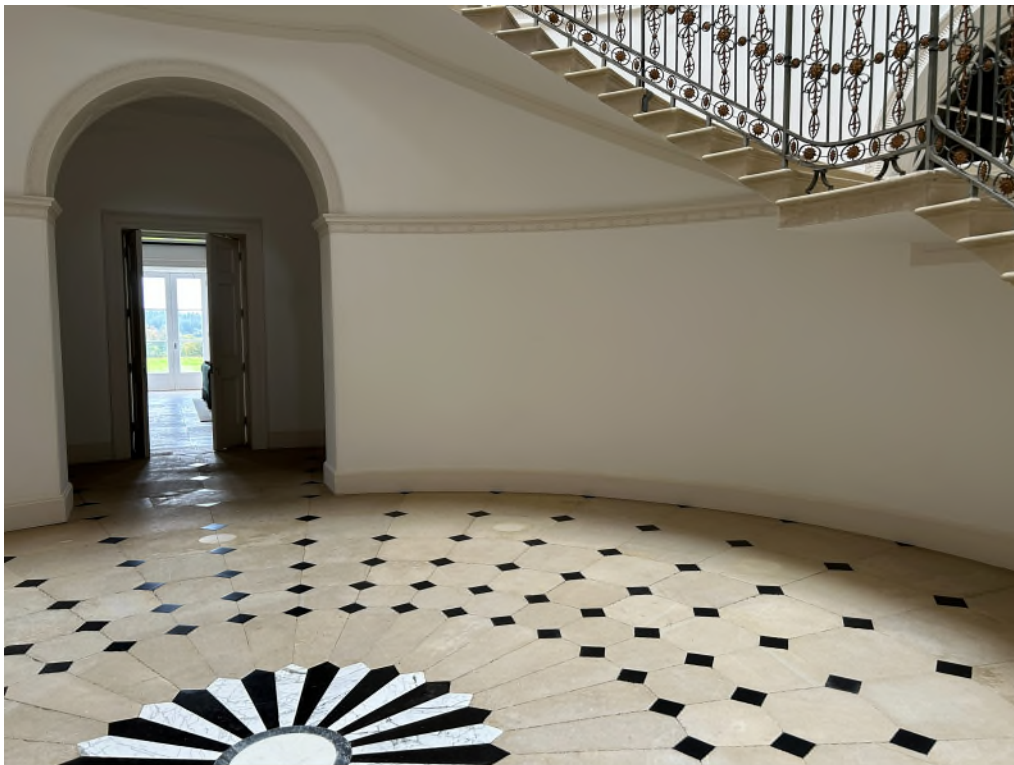
Figure 75: R.G.21, Main Staircase, stone floor & doorway to Garden Room
