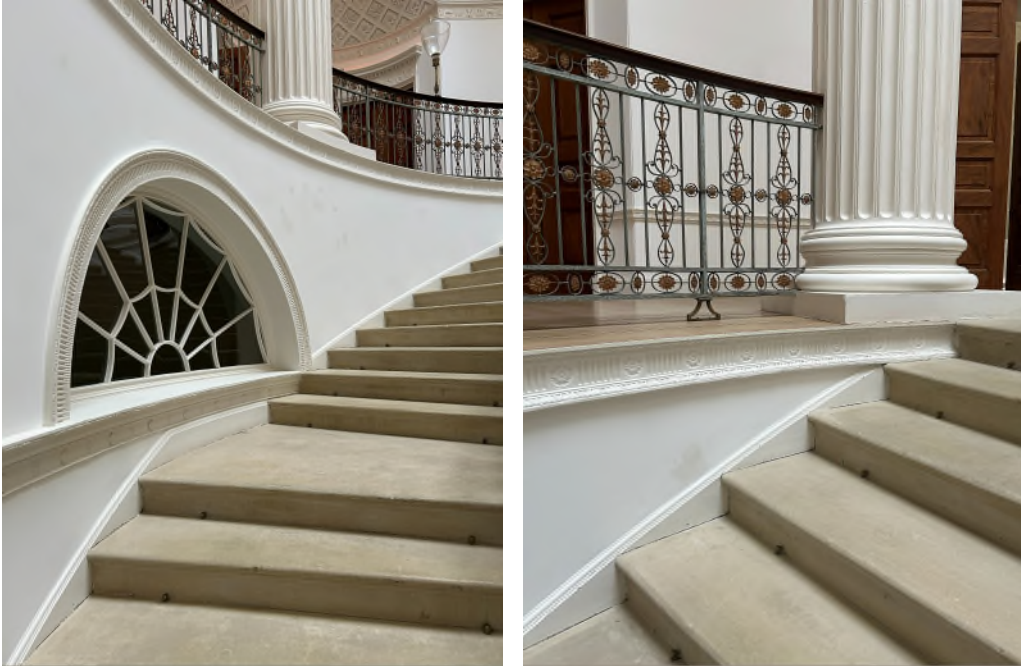
Figures 76 & 77: R.G.21, Main Staircase, lunette window onto East Ambulatory, railing detail
