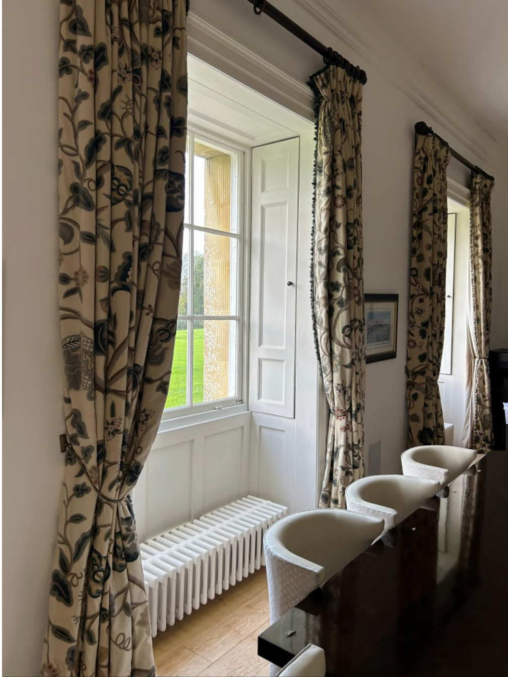
Figure 23: R.G.07, Office: panelled window shutters
