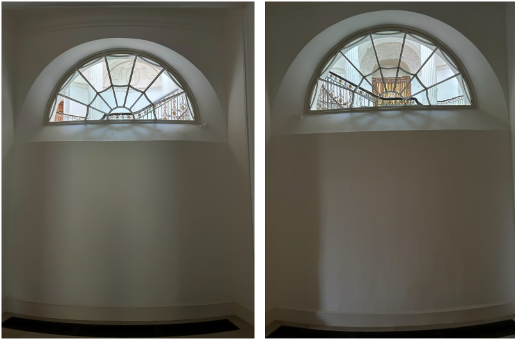
Figures 64 & 65: R.G.19, East Ambulatory (proposed R.G.20), lunette windows looking onto the Main Staircase
