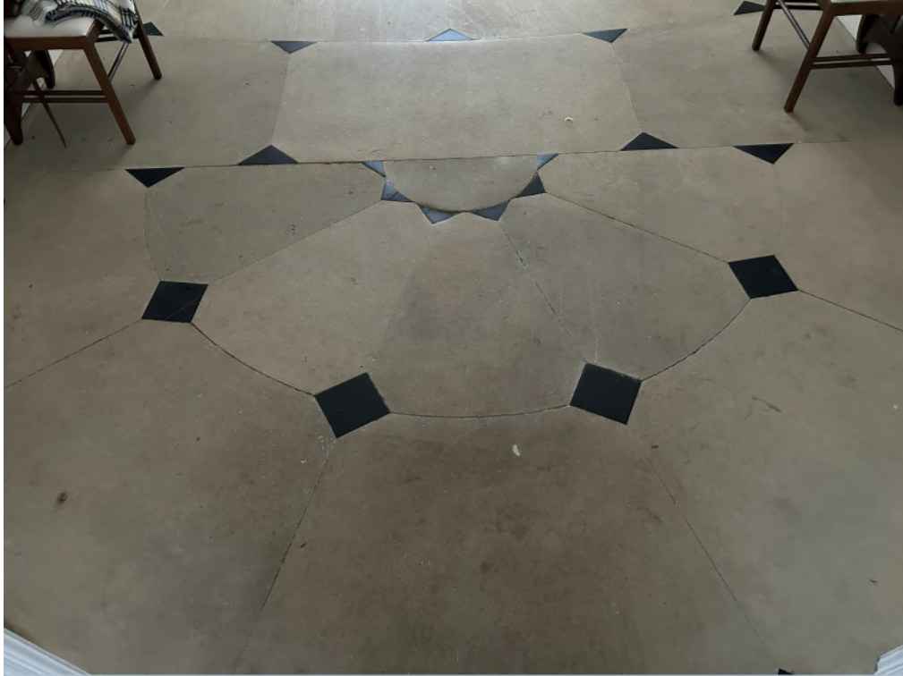
Figure 58: R.G.18, North Lobby (proposed R.G.19, North Lobby), stone floor pattern
