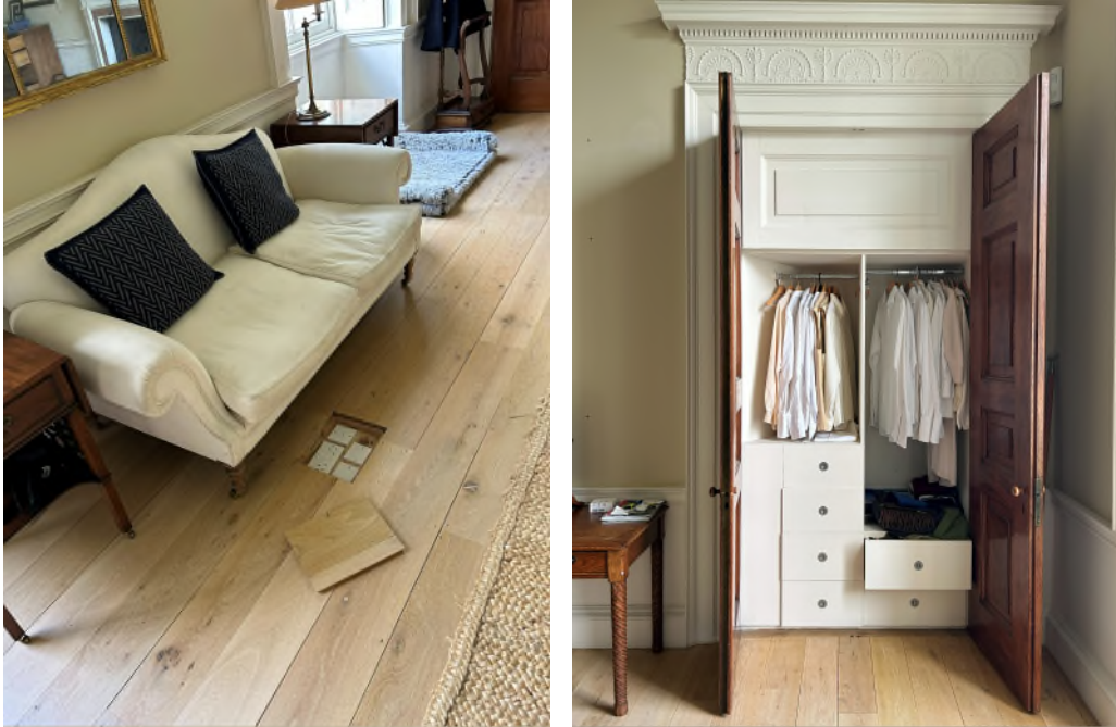
Figures 108 & 109: R.1.07, Bed 2 (Main Bathroom)
