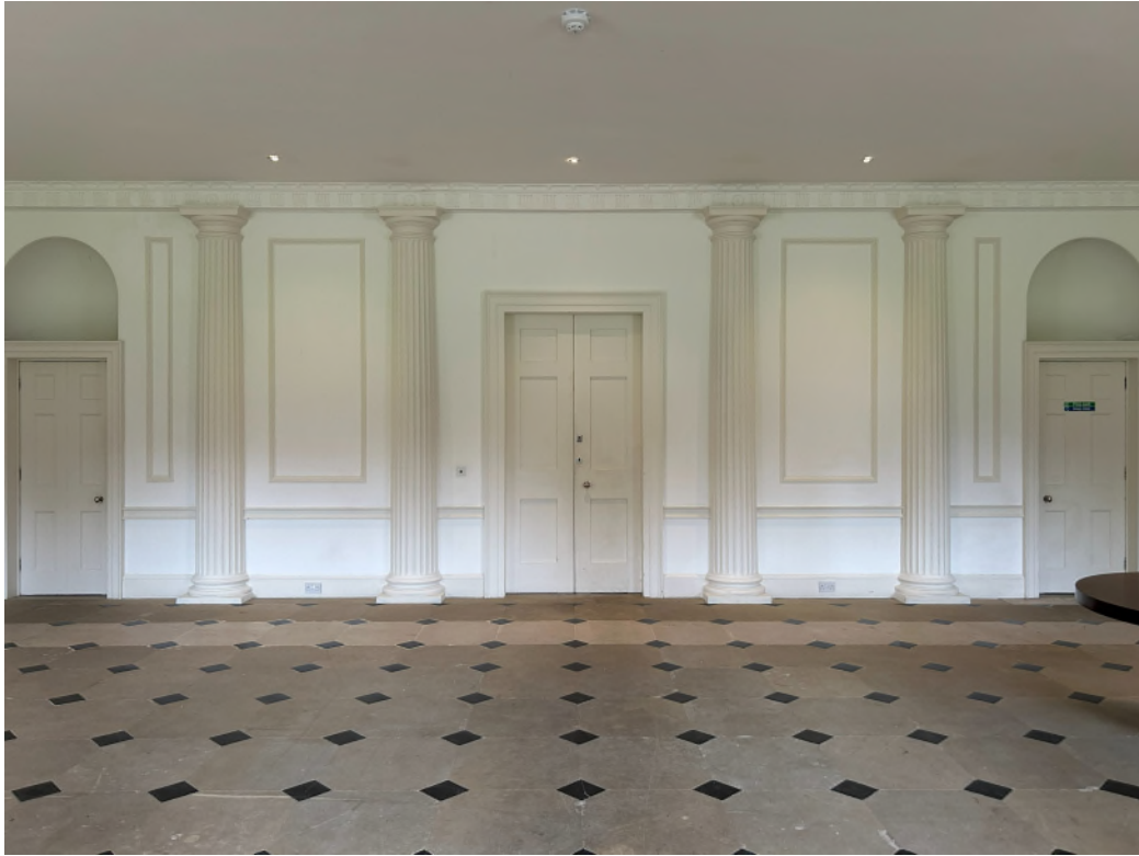
Figure 1: R.G.01, Hall: door to North Lobby
