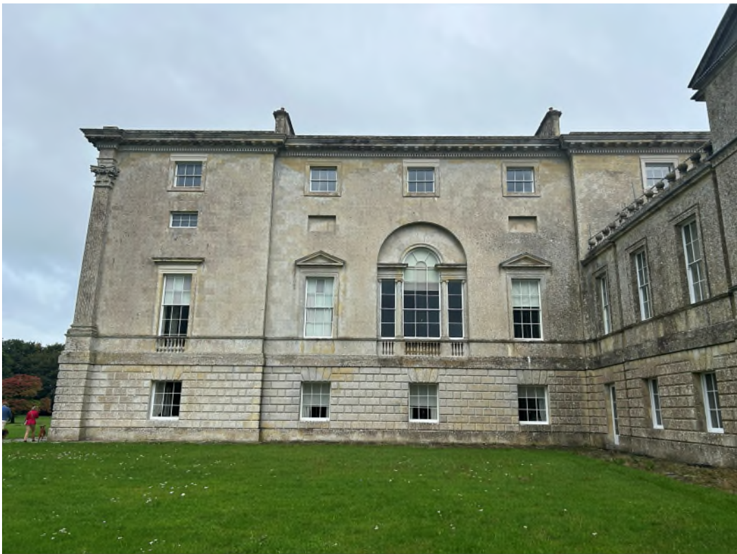
Figure 140: External, East façade
