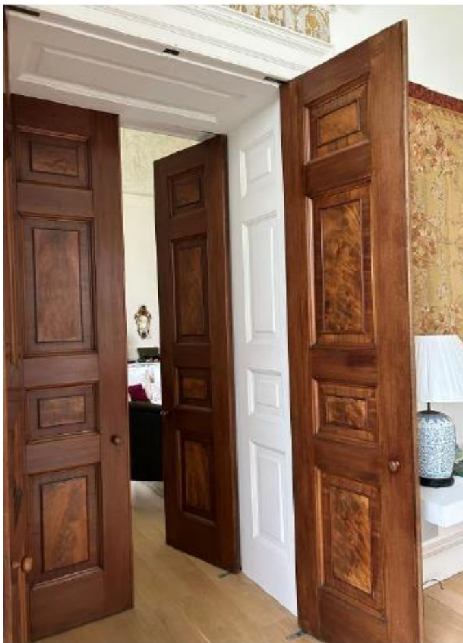
Fig.9 Panelled doors and reveals to the Dining Room
