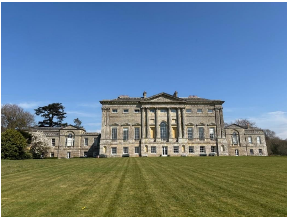
Fig.5 South façade of the house
