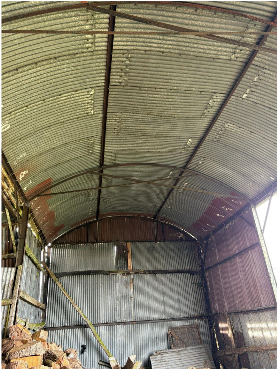
General View of Roof Structure
