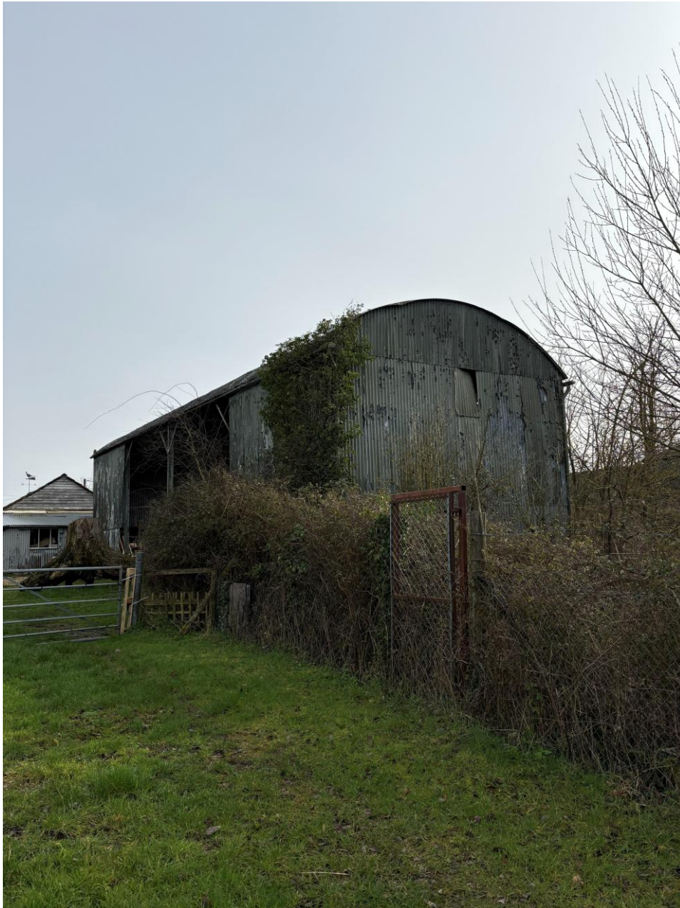
General View of Building West Elevation
