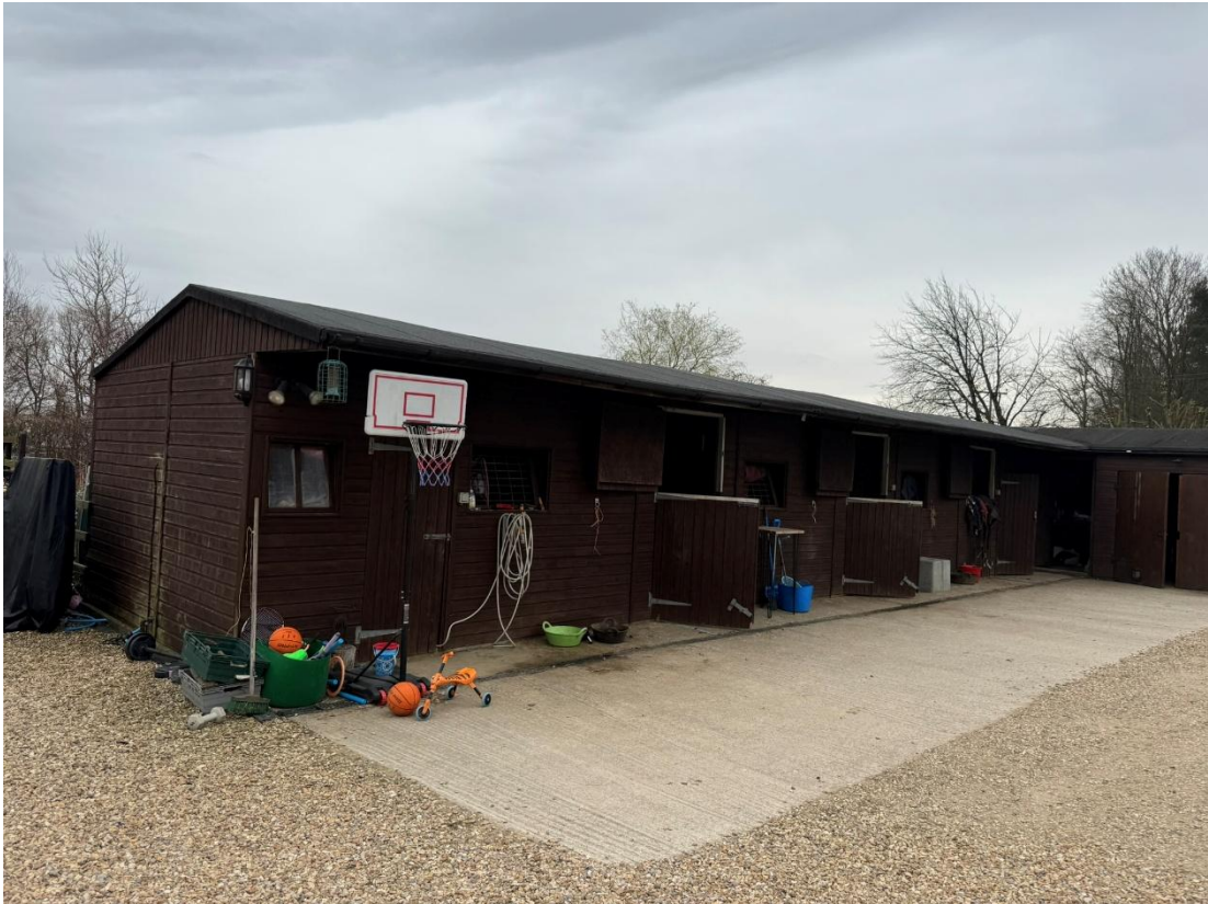
Plate 5: Front elevation of stable block
