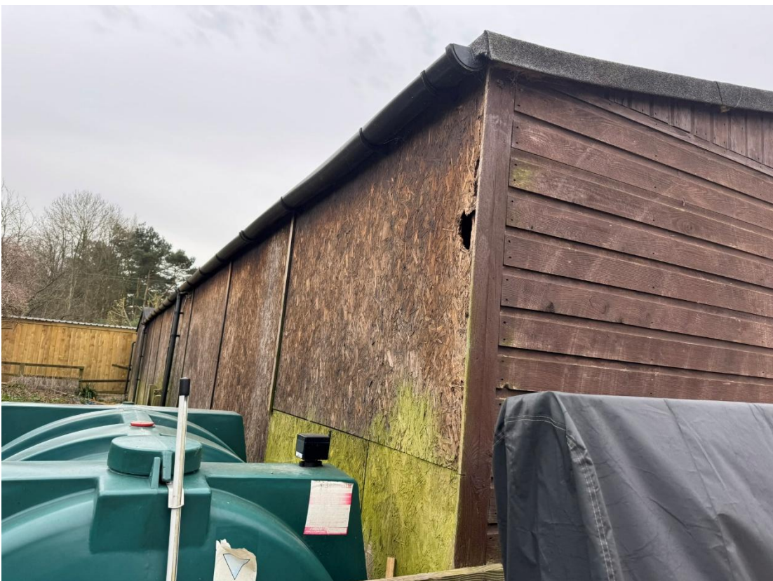
Plate 6: Rear elevation of stable block
