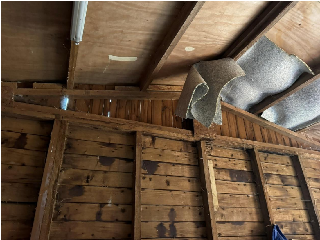
Plate 7: Interior view of stable block showing single skin timber and ply roof
