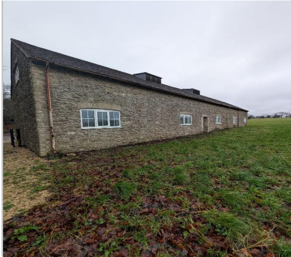
Figure 5 - east elevation of the building.
