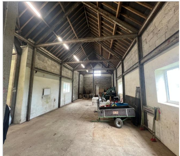
Figure 14 – interior of the building.
