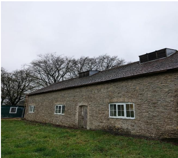
Figure 9- east elevation of the building and adjacent grassland.
