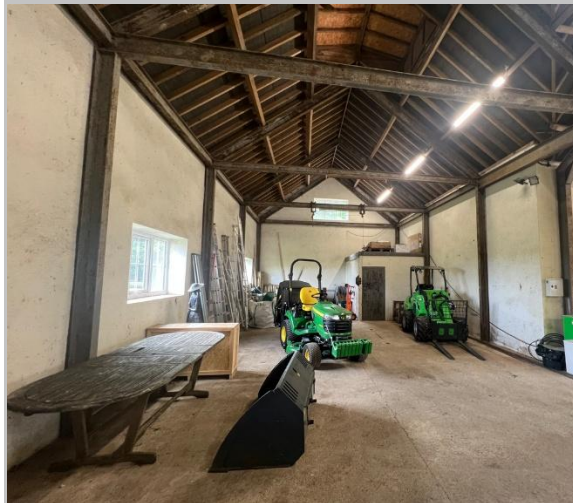
Figure 15 – interior of the building.
