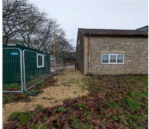
Figure 6 - southern elevation of the building.
