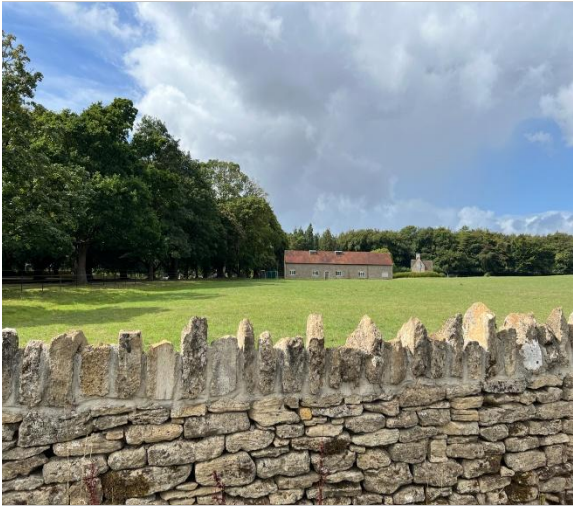
Figure 17 – stone wall and overview of the field from Blackberry Lane to the south.
