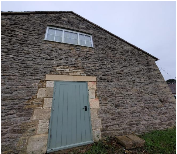
Figure 10 - north elevation of the building.
