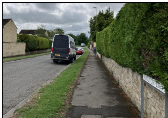
Image 3.2 Pedestrian Footways on Moulton Drive
