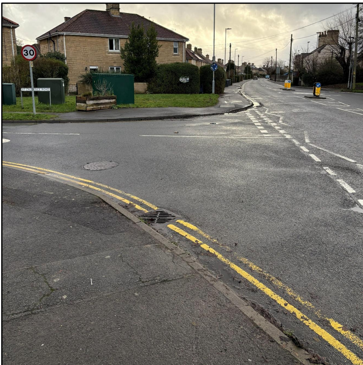
Photo 2.1 Crossing at St Laurence Road / Trowbridge Road junction
