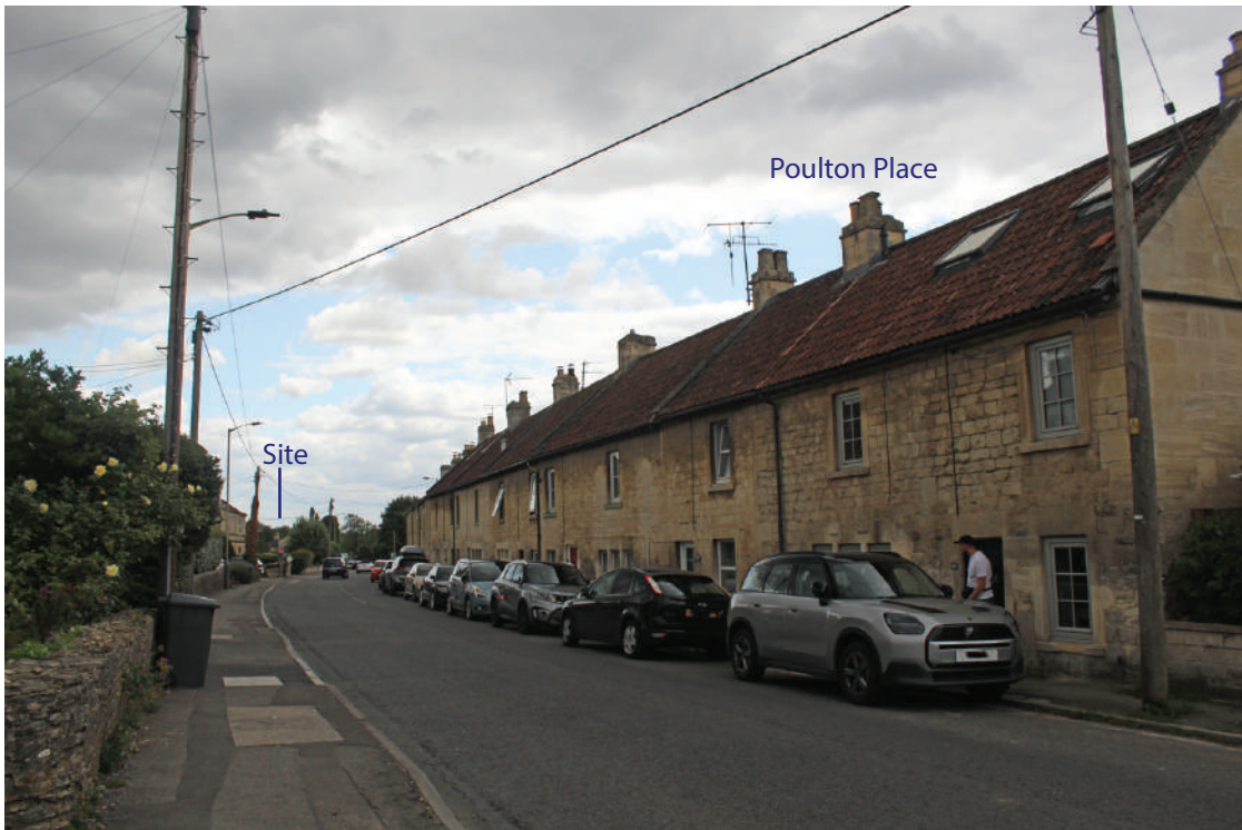
Photo 21: Travelling south-east down Trowbridge Road
