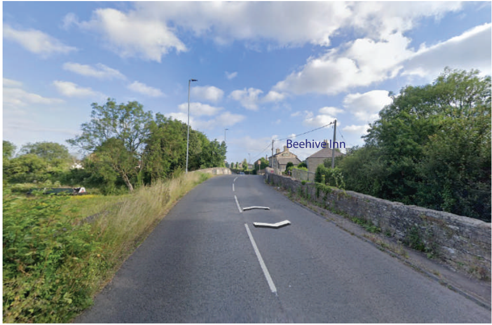
Photo 14a: The approach to Widbrook Bridge on the Trowbridge Road (courtesy Google Earth)
