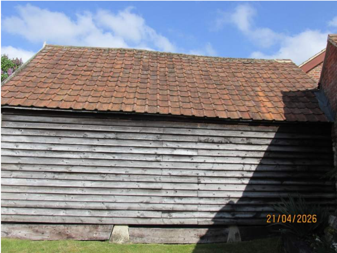
Building 2 – External view of south elevation
