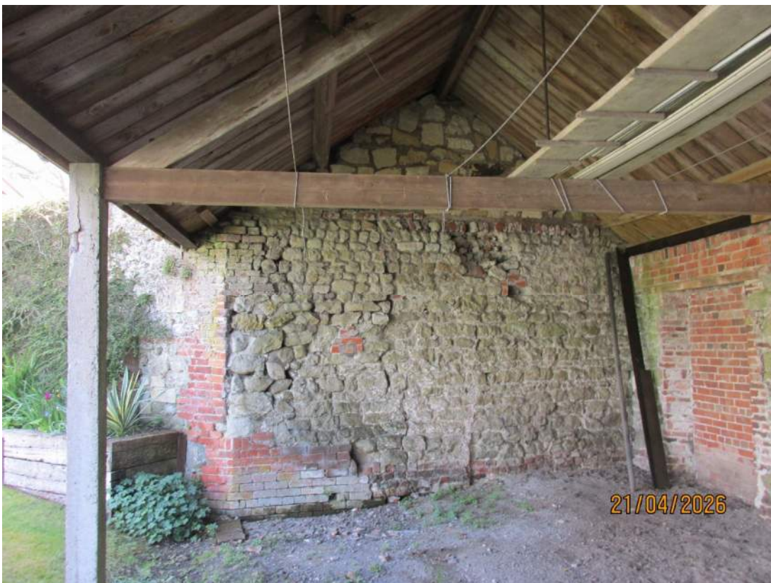
Building 1 – View of end gable (party) wall of Store
