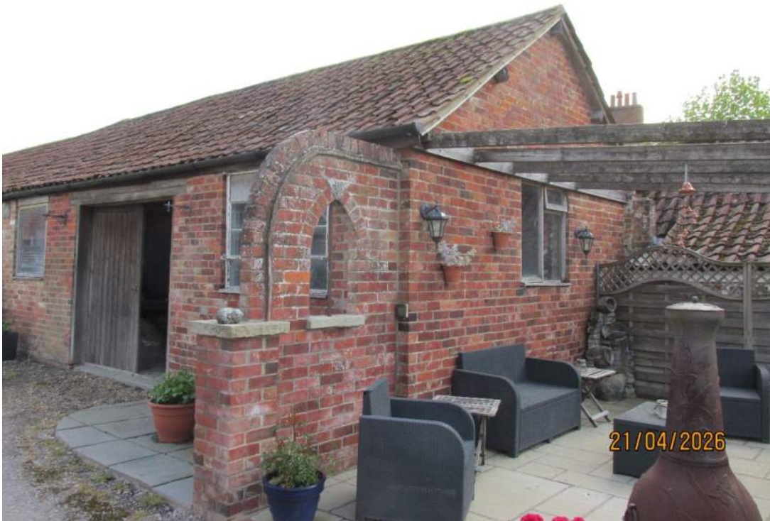
Building 1 – External gable elevation viewed from south west
