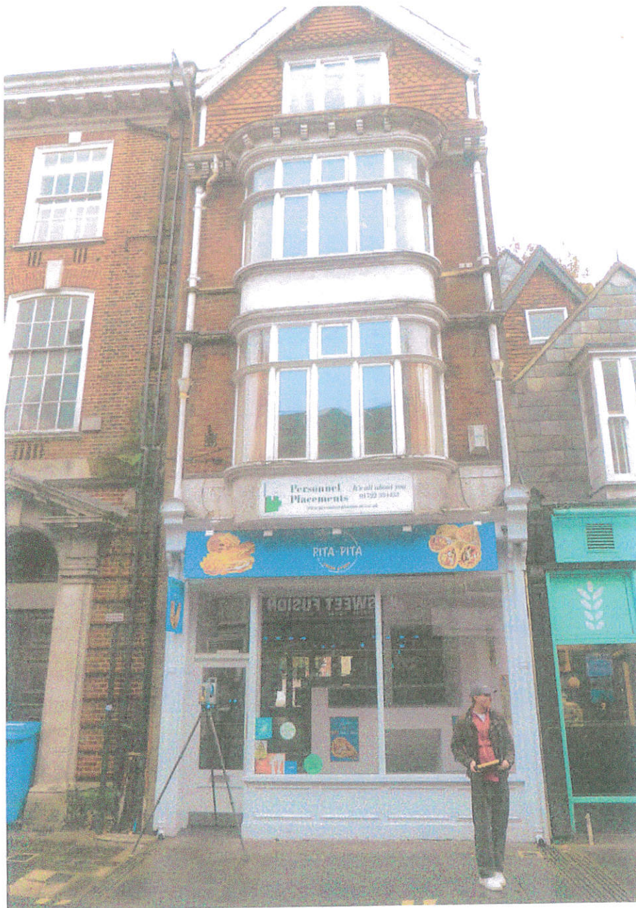
Directly opposite No12 showing whole facade
