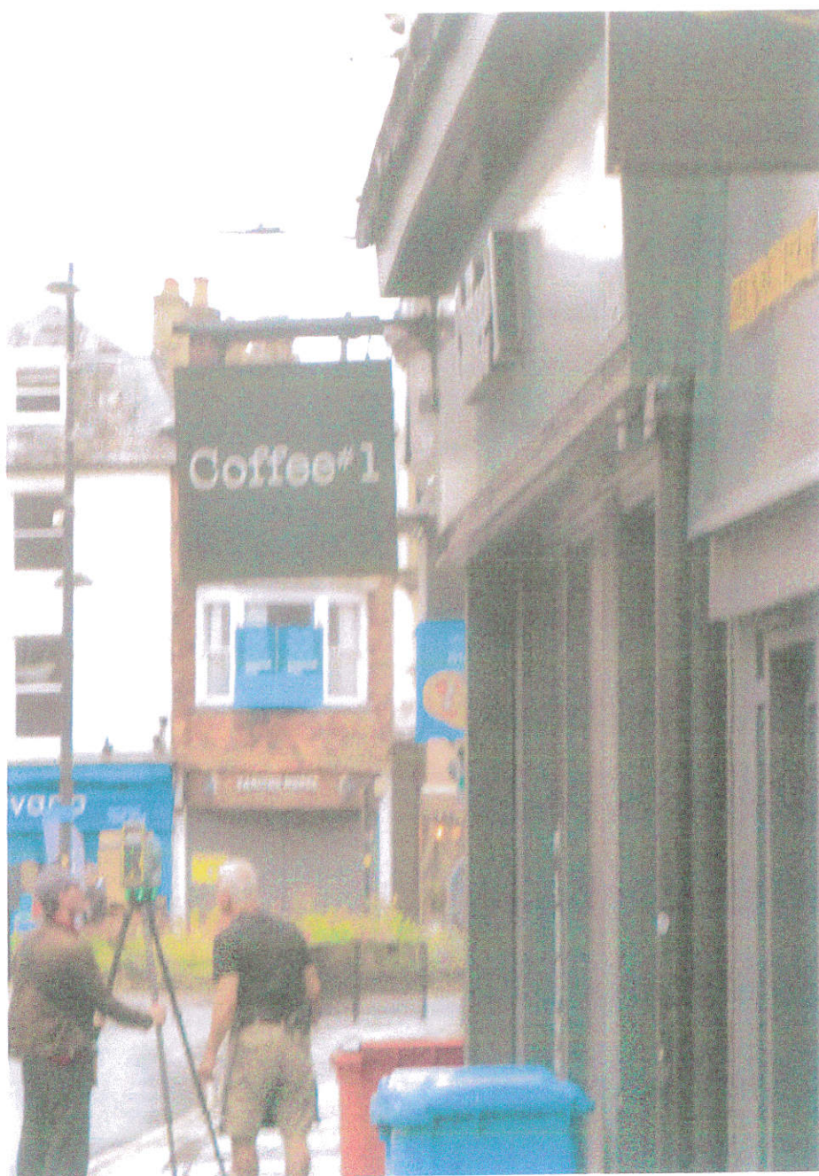
Enlarged view of premises from same side as the Poultry Cross showing 50% of the fixed projecting sign is obscured
