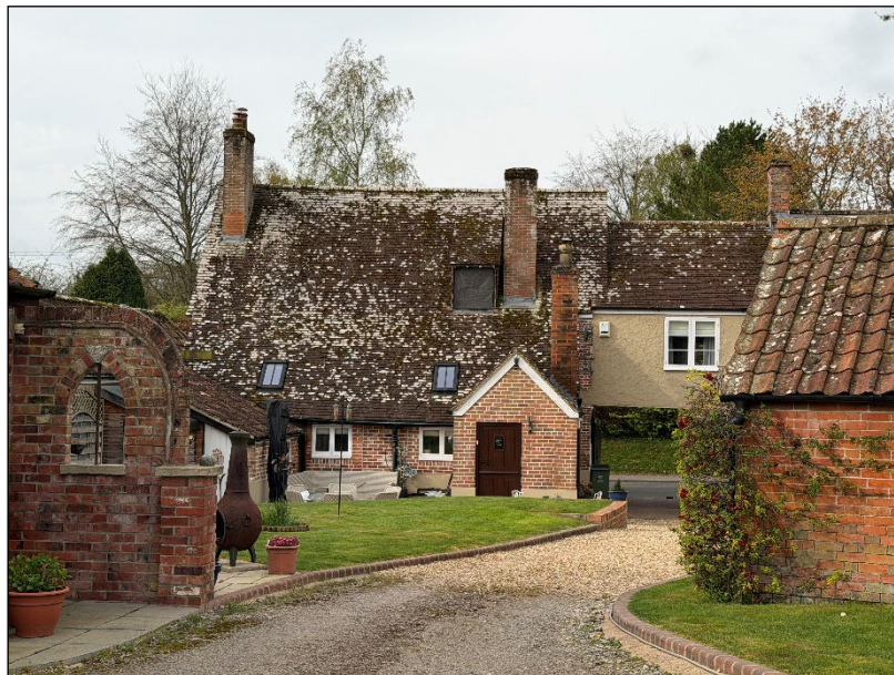
Image 17: No. 69 High Street, rear elevation
