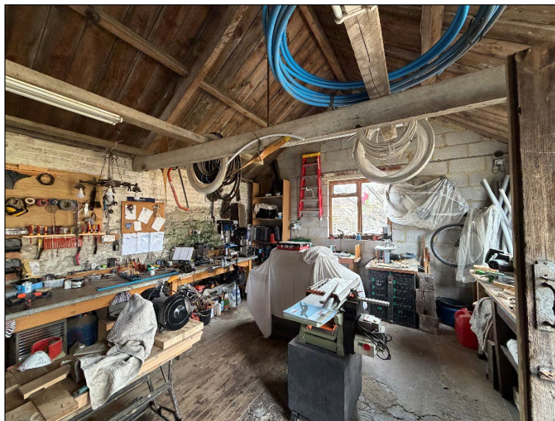
Image 15: Internal view showing replacement roof structure
