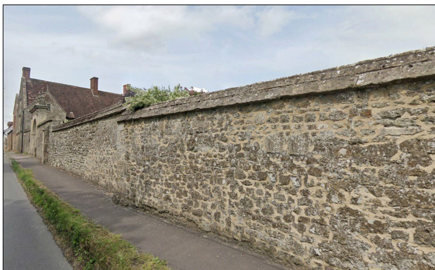
Image 19: Boundary wall to West Lavington Manor
