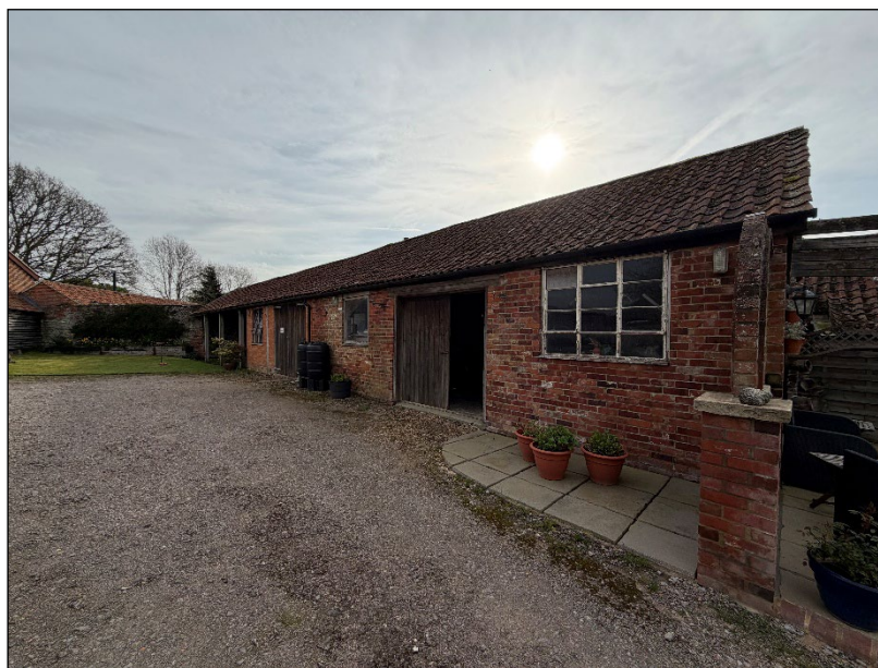
Image 13: Outbuilding viewed from southwest
