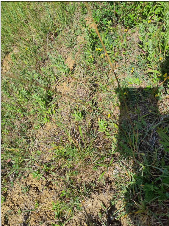
Site Walkover 26.06.2025: Cracks due to possible desiccation located on the slope (Facing North)
