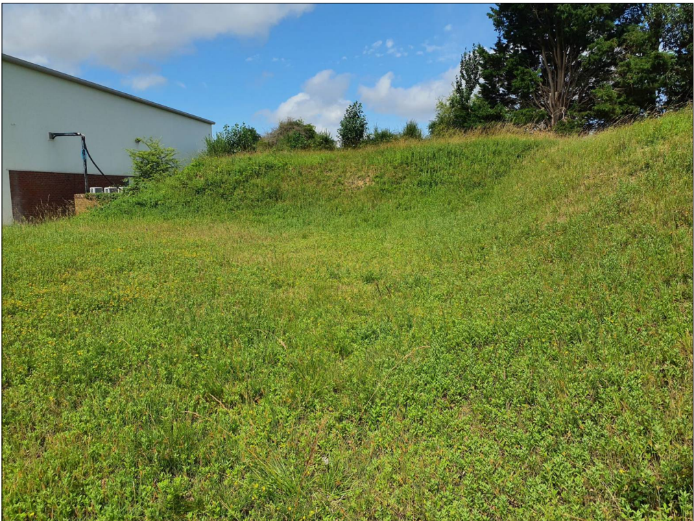
Site Walkover 26.06.2025: Slope located in the proposed location (Facing Northwest)
