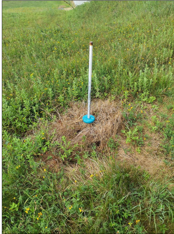
Site Walkover 26.06.2025: Metal pipe around top of the slope (Facing North)
