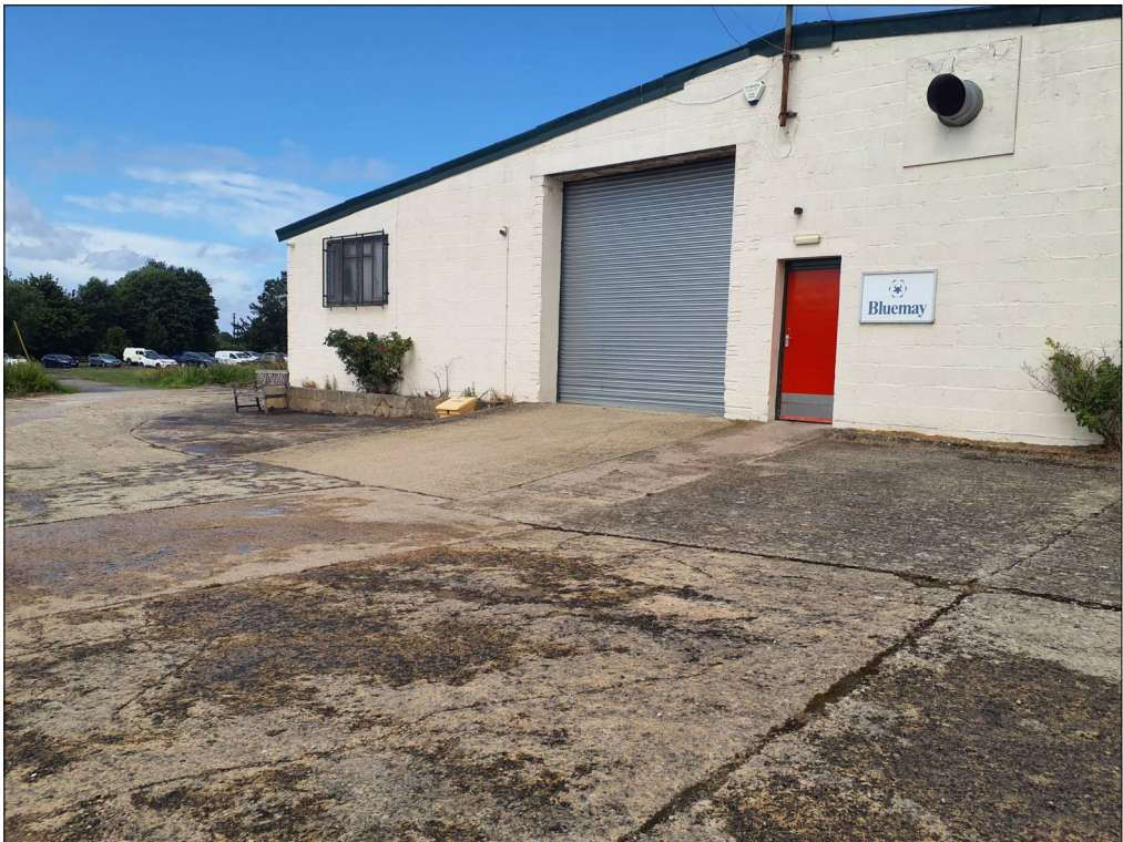
Site Walkover 26.06.2025: Existing unit 2 (Facing Northeast)
