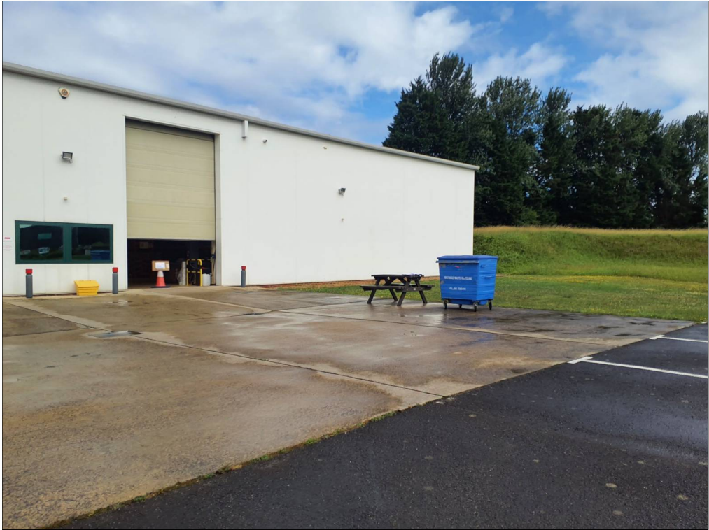
Site Walkover 26.06.2025: Existing unit 1 (Facing west)
