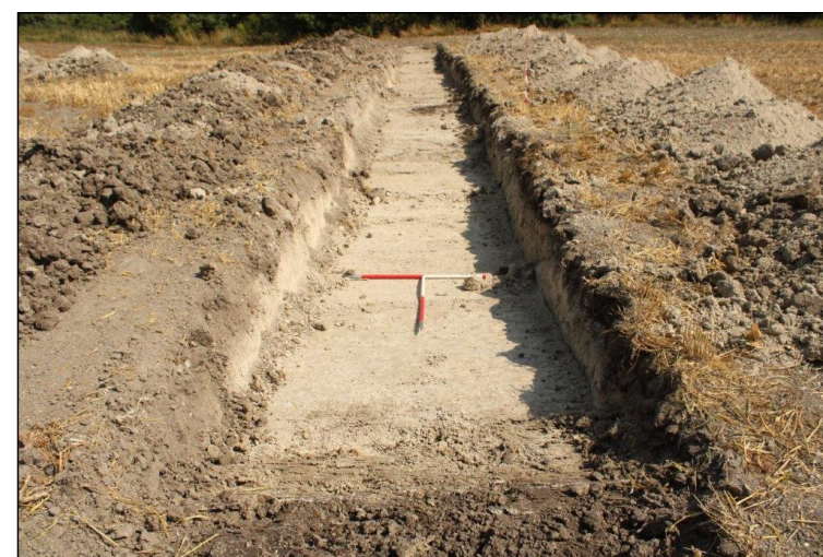
Figure 6.3: Trench 2, view north-east, 2 x 1m scales
