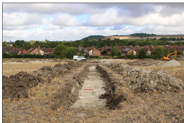
Figure 6.4: Trench 4 view northwest, with 2 x 1m scales
