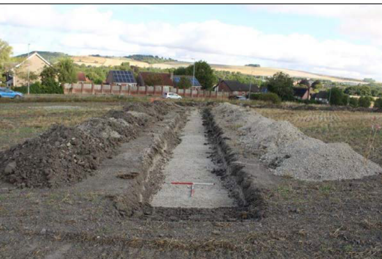
Figure 7.7: Trench 15, view north, 2 x 1m scales
