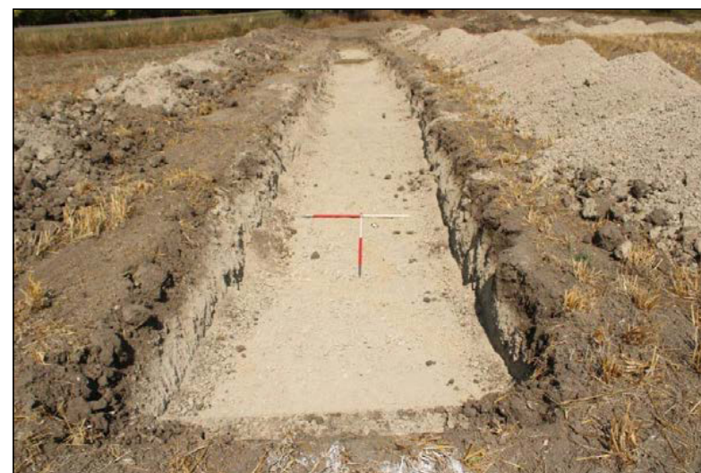
Figure 7.2: Trench 11, view north, 2 x 1m scales
