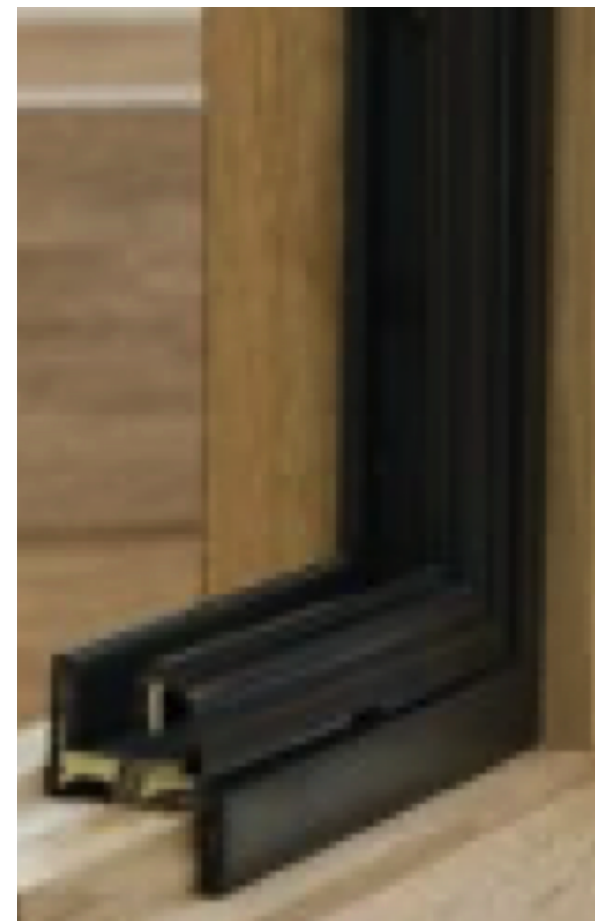
View of metal window in timber frame
