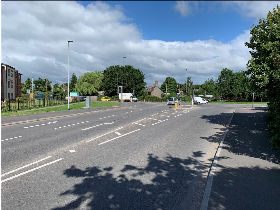
Photograph 3.2: View to the north along Windsor Drive to the A361 London Road/Windsor Drive Signal Controlled Junction
