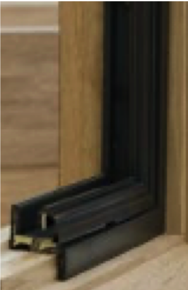
View of metal window in timber frame
