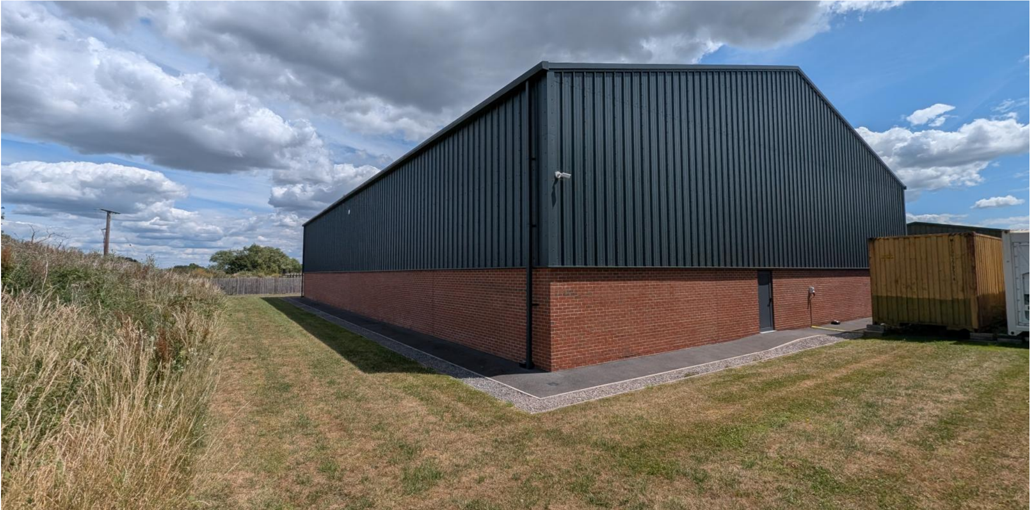
Photo 4: Oblique north / west facing view of Tinplate's warehouse. The portal framed building is constructed out of brick with profiled metal sheeting to the upper wall and roof.
