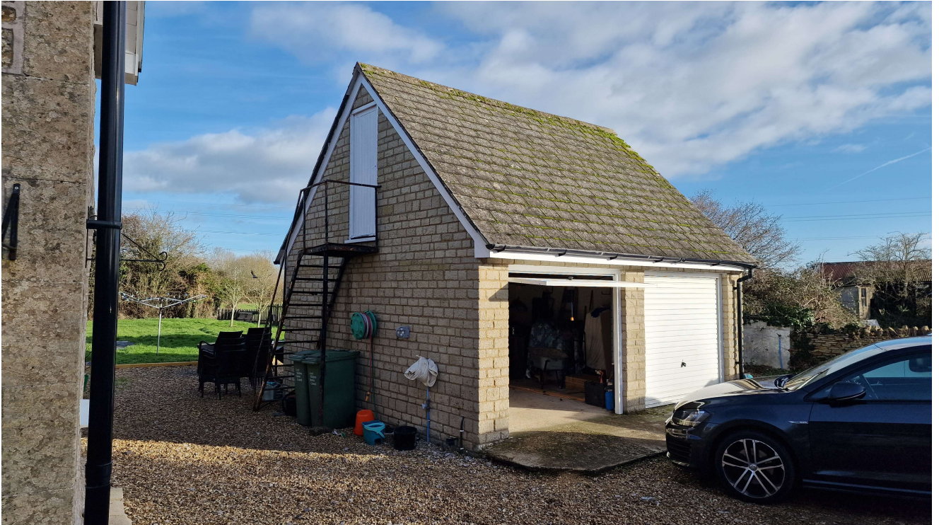
Front and west side elevation of garage
