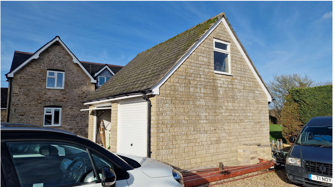
Front and east side elevation of garage
