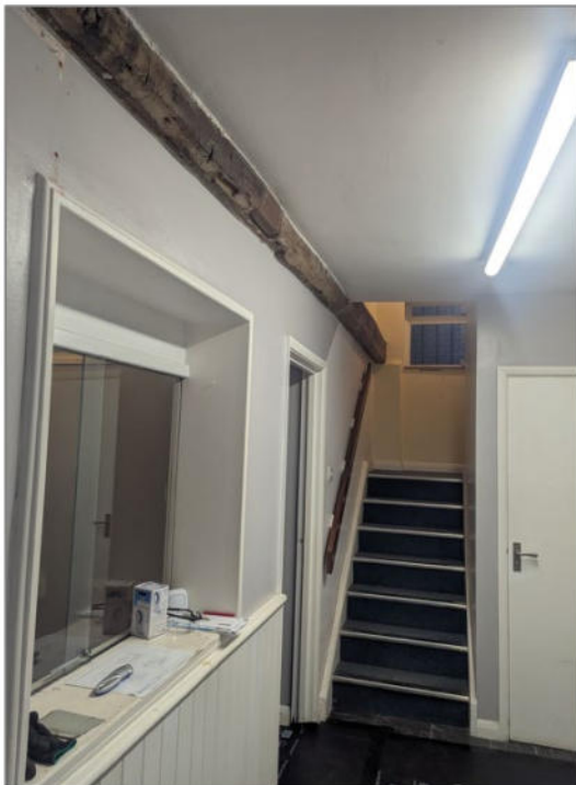
Figure 4 - Existing ground floor entrance
