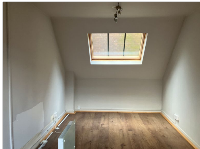
Figure 7 - Existing second floor meeting room
