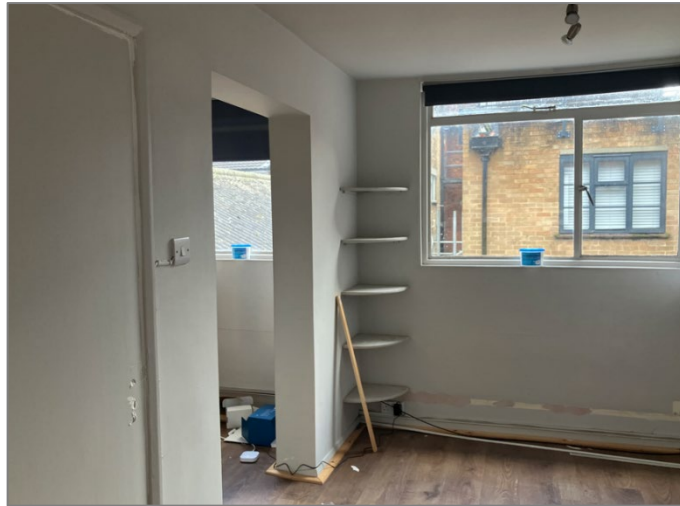
Figure 6 - Existing first floor office
