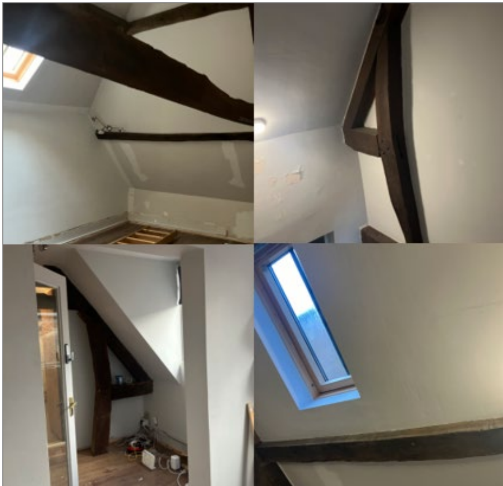
Figure 23 - Exposed beams and trusses
