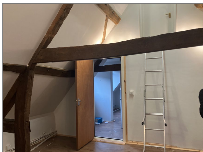
Figure 8 - Exposed historic beams and trusses
