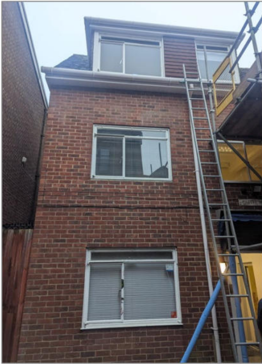
Figure 2 - Existing front facade
