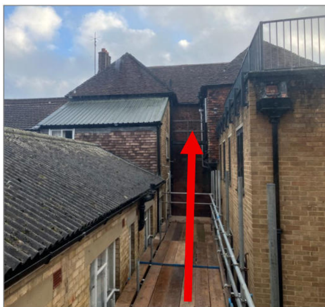
Figure 24 - Intervening buildings between front facade and Castle Street
