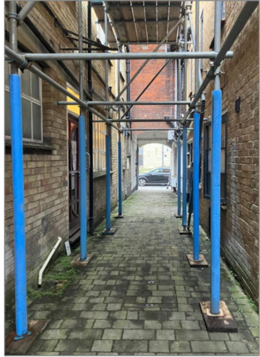
Figure 3 - Existing alleyway off Castle Street
