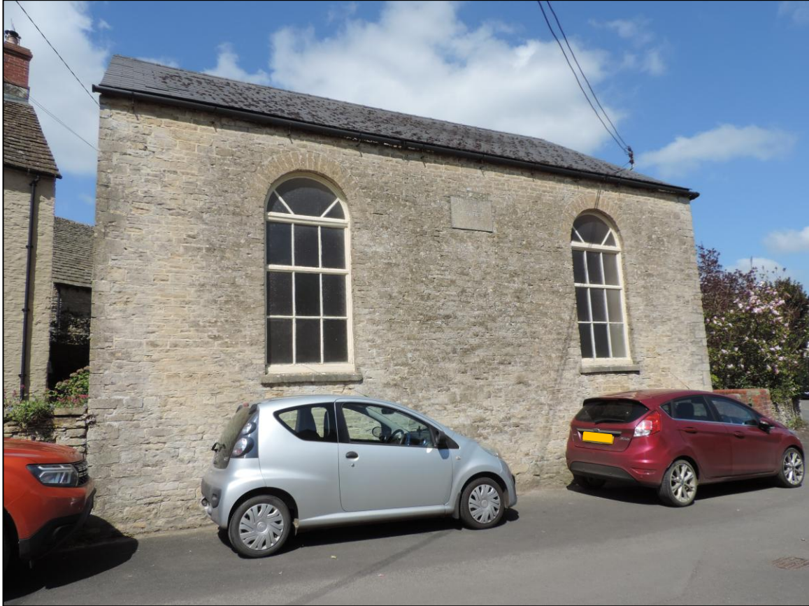
Photo 5 Former Sherston Methodist Chapel, Grove Road southeast elevation, fronting Grove Road.
