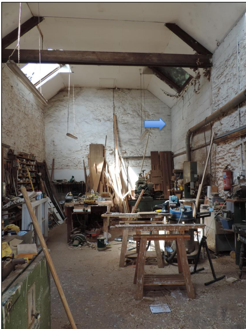
Photo 10 WSW facing view of interior of NDHA-B 19th century stone building with floor to ceiling infill evident to the right- indicated with the blue arrow.
