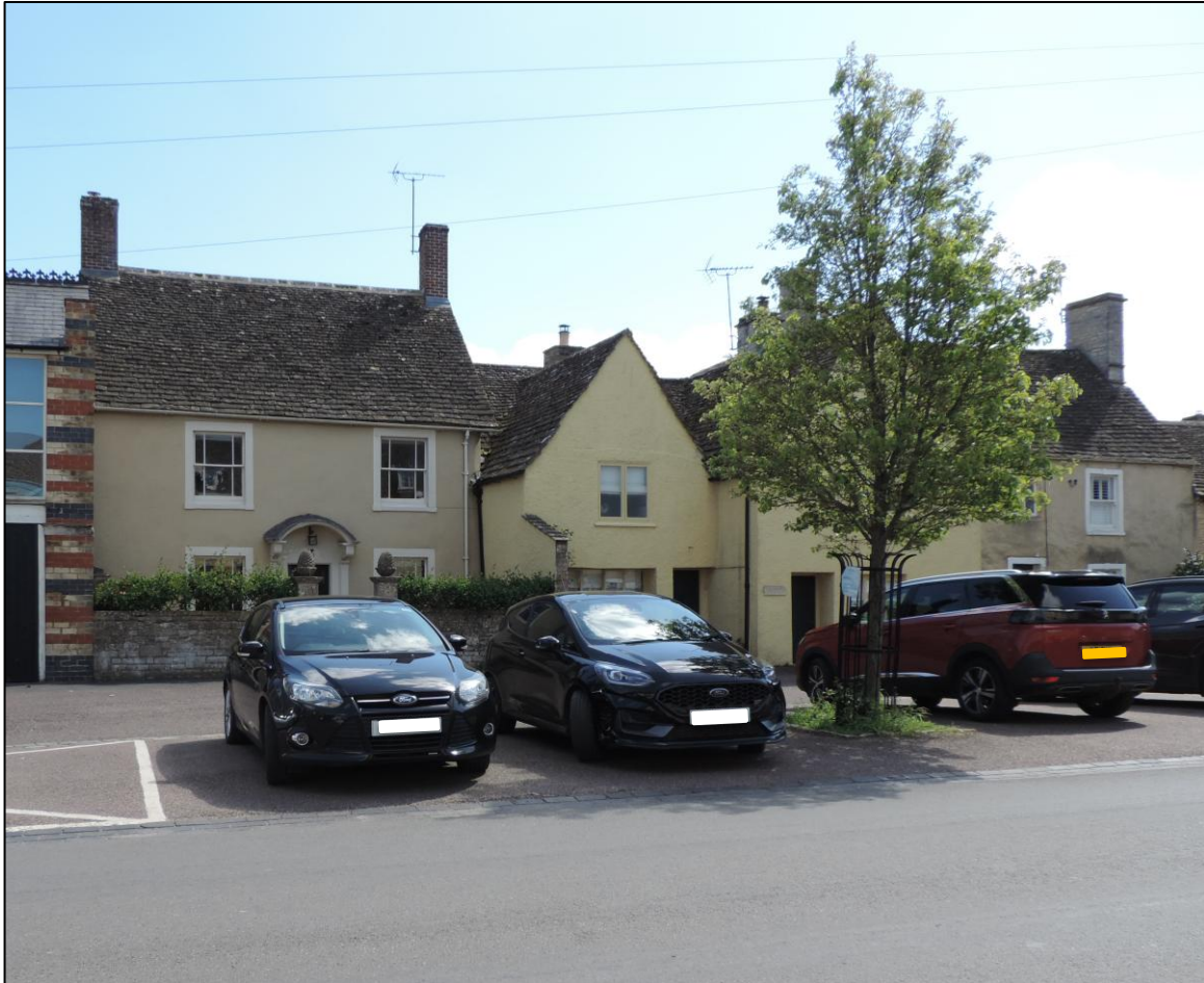
Photo 4 East facing view of grade II listed The Pines, No. 16 High Street, principal elevation (left)
