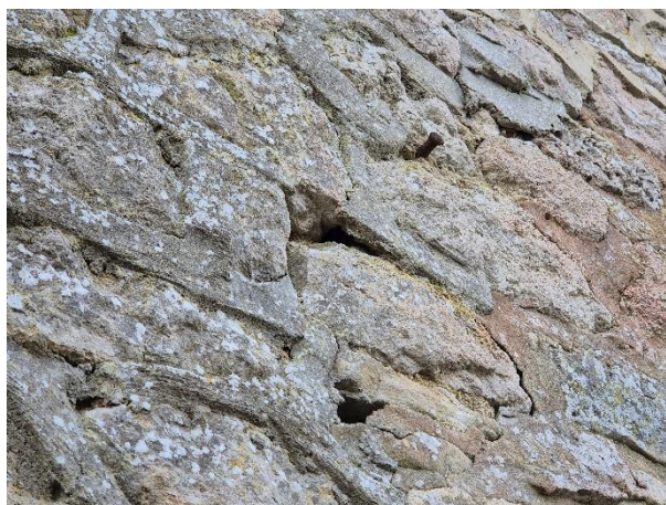
Photo 6: Missing mortar
