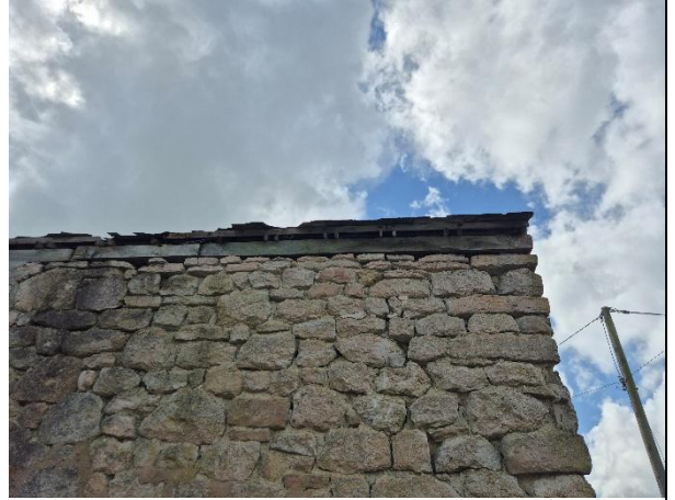
Photo 10: Missing bricks and timber provide access
