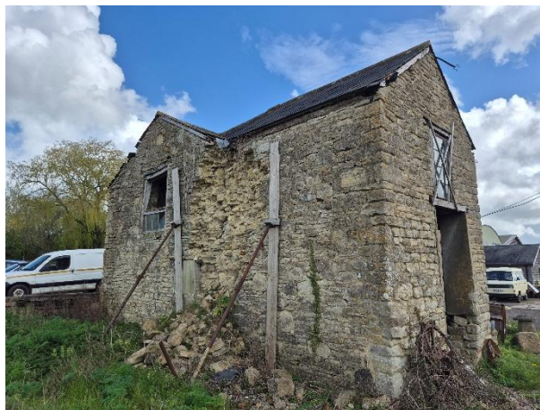
Photo 4: Partially collapsed eastern aspect
