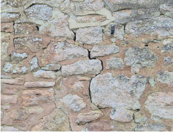
Photo 9: Missing mortar potentially leading to a cavity
