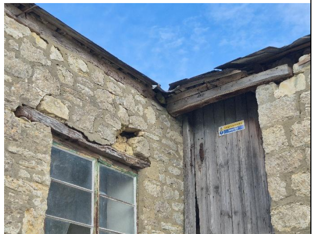
Photo 12: Gap around the wooden window frame and a gap above the door caused by missing timber provide access
