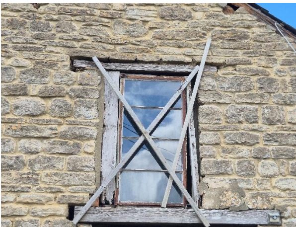
Photo 11: Gaps around the wooden window frame on the southern aspect provide access into the building
