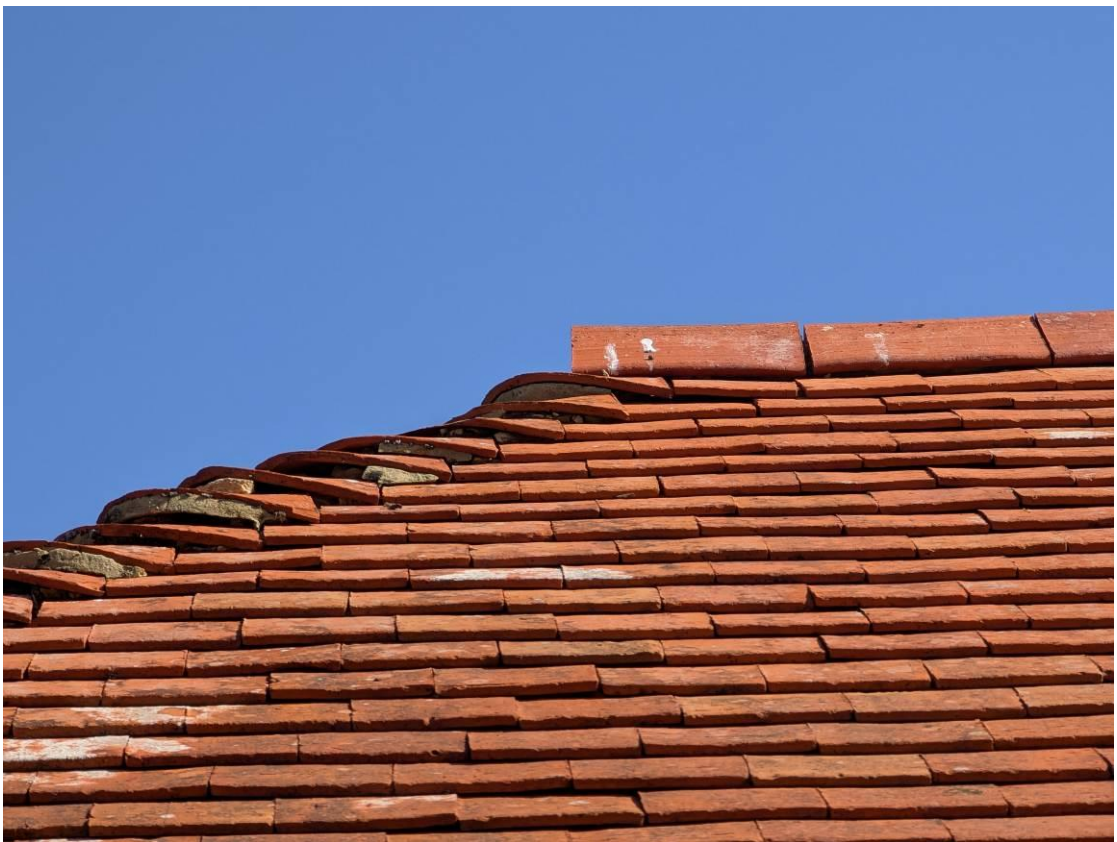
Photo 3/4 The Old Livery, (south aspect) clay roof tiles with access gaps
