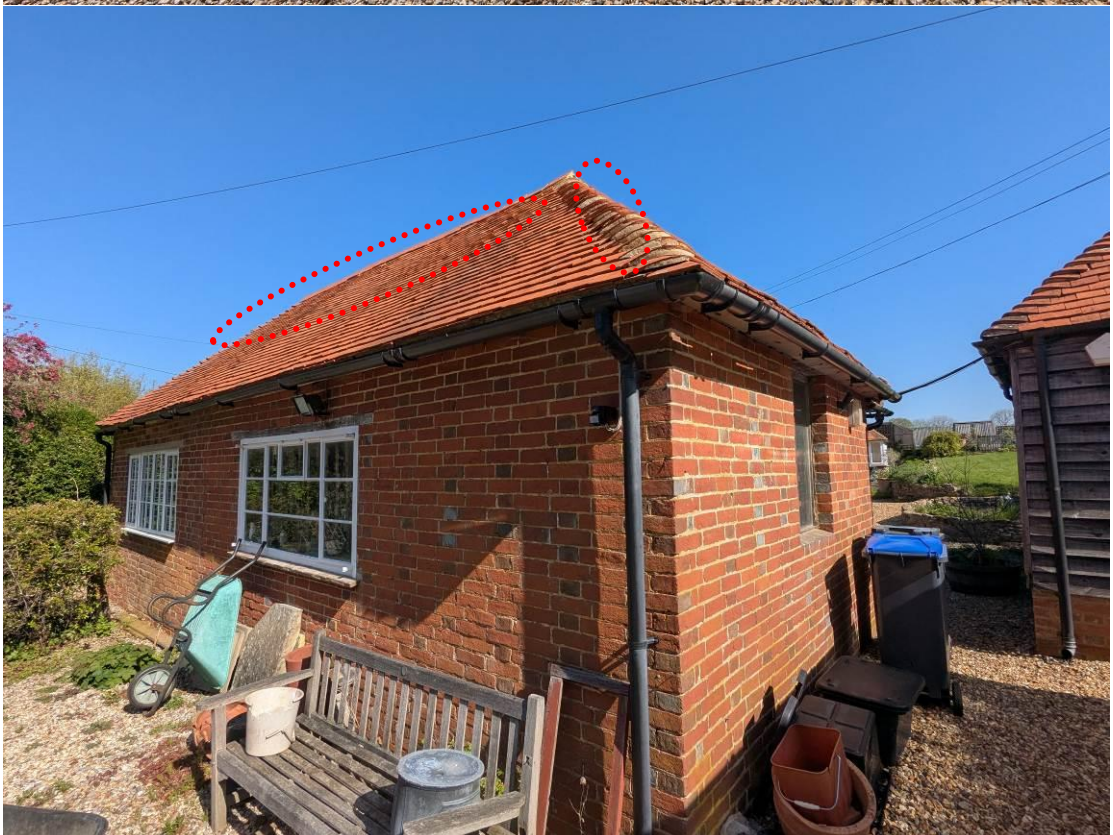
Photo 1/2 The Old Livery, north and south aspect) potential roost features –clay roof tiles.
