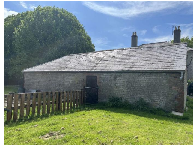
Photo 2: North elevation of B1
