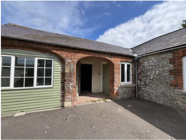
Photo 1: West elevation of B1
