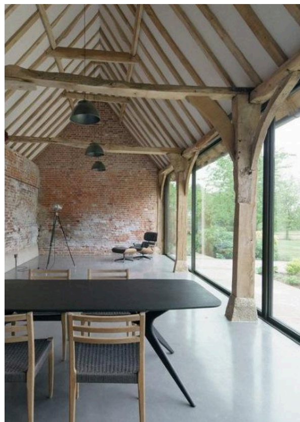
Fig 7. An example of where glazing on the outside of the original columns maintains the original appearance of the barn
