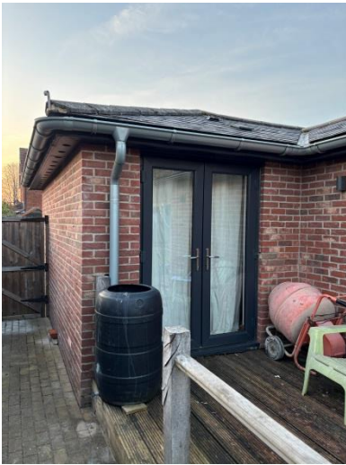
Image of the Existing South East Elevation, where the proposed extension will be constructed
