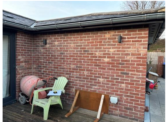
Further Image of the South East Elevation. Image shows the hipped roof to be removed and replaced with a flat roof
