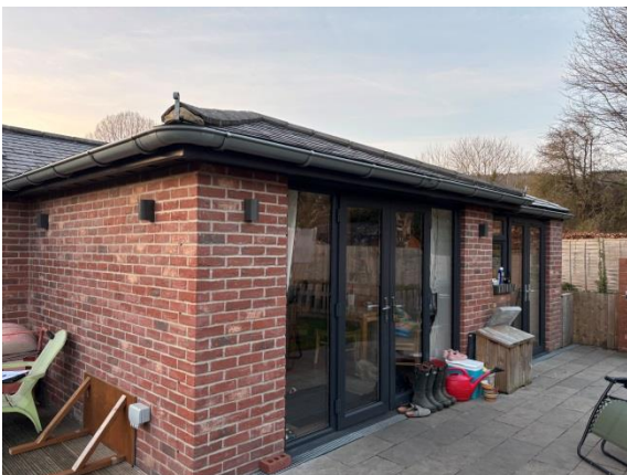
Further Image of the Existing South East Elevation which will receive cladding to the walls, the pitched roof will be removed and replaced with a parapet and flat roof.
