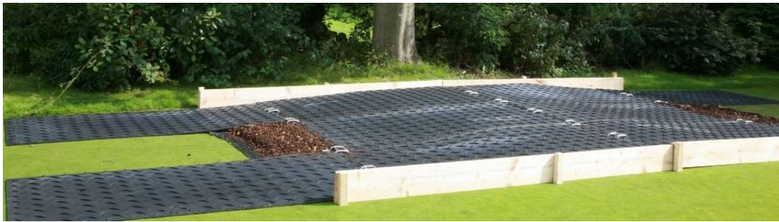
Figure 4: Example of proprietary, inter-linked ground protection boards used as tree root protection.
