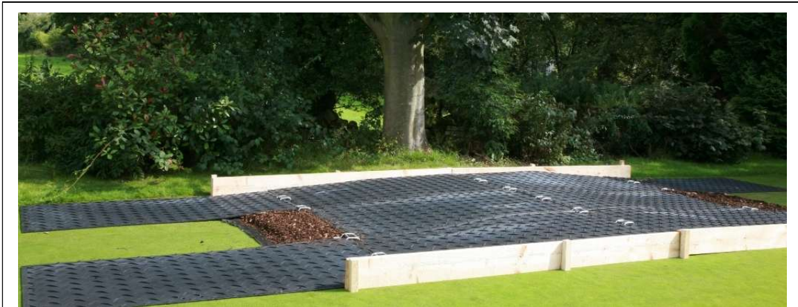
Figure 4: Example of proprietary, inter-linked ground protection boards used as tree root protection.
